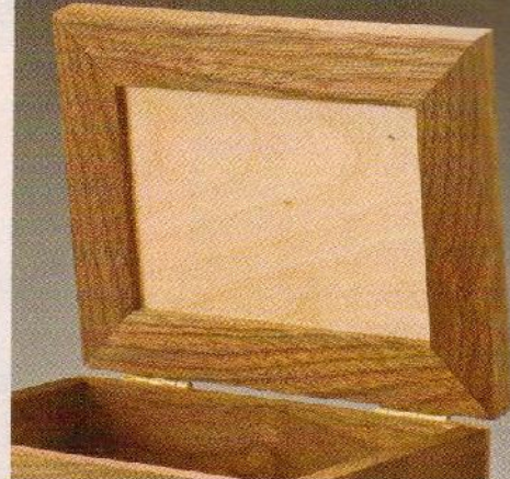
Use hinges to attach the framed lid to the box sides.
