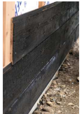
The exterior cladding will be done with yaki sugi (charred cedar boards). It is said that creating a carbonised layer on the surface makes it stronger against rot and insects (above)
