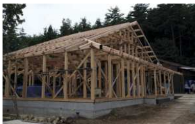
The assembled timber frame structure (left), which took three days to assemble. The current state of the workshop (above). Work continues on the roof & exterior
