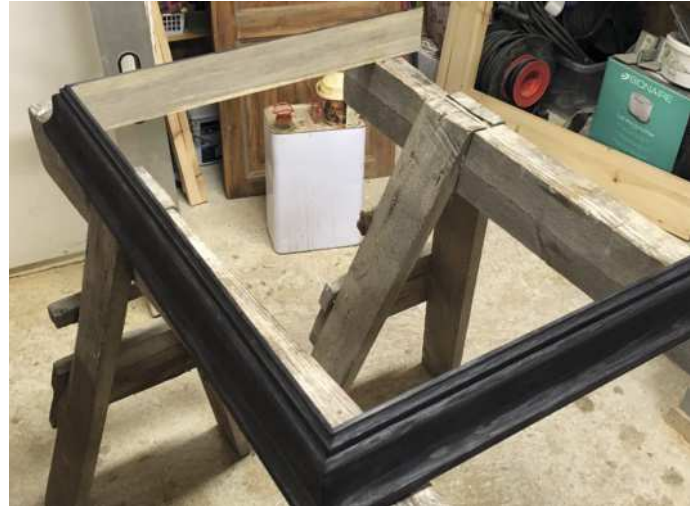
Dry-fitting the newly assembled cornice (above), stained and oiled (right)
