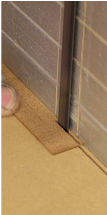
The second cut (above) creates the square line. Keeping fingers a little behind the blade and a constant gentle pressure prevents bloodshed and reduces splinters
