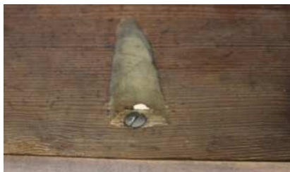
A screw well (above) on an 18th Century Virginian table. Note the maker dug the well too deep and pierced the outside face of the table apron. Two finished screw wells (right) on adjoining aprons of the sideboard table, ready for screws and top attachment
