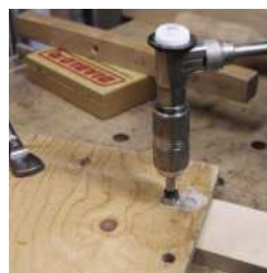
A bubble level (above) taped to the brace aids in drilling plumb holes. If the bench does not have any holes, drill two to match the dowels on the bench hook (right). The two-way fixture can be made new or modified from an existing one, with dowels holding the jig for pull sawing
