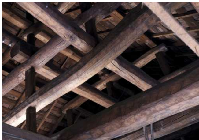
The distinctive marks (above) left by hand-tools can be seen on the beams of traditional houses. Looking up at them makes one marvel at the skills of the carpenters of the past, who only had hand tools to work on such sizeable materials
