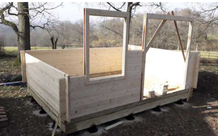
The whole thing goes together like Lego, and ready for roofing (right)
