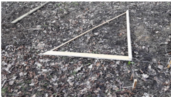
The 3-4-5 triangle in use. I pegged out the outline of the shed with some string (above). This helped with positioning of the shed and with placing the concrete slabs for the frame supports later. The doorframe fixed up square (right)
