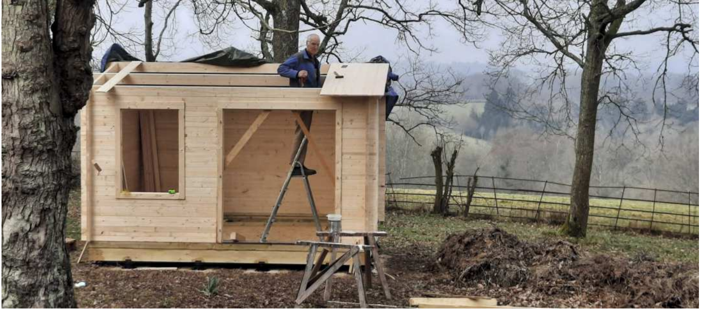
Installing the 15mm tongue and groove roof boards. The long and thin nails provided when in beautifully, without bending, and have good grip. Beginnings of the base construction (right). The green stains are an end-grain protector called End Coat from Osmose
