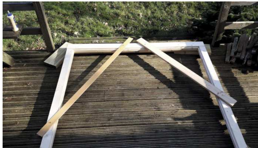
The 3-4-5 triangle in use. I pegged out the outline of the shed with some string (above). This helped with positioning of the shed and with placing the concrete slabs for the frame supports later. The doorframe fixed up square (right)
