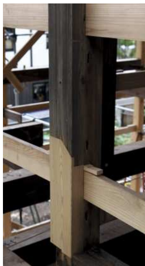
The second-floor beams I was in charge of. Repairing the old materials, working on the curved beams, marking and cutting out the new materials. This part is an extended area of the original structure
