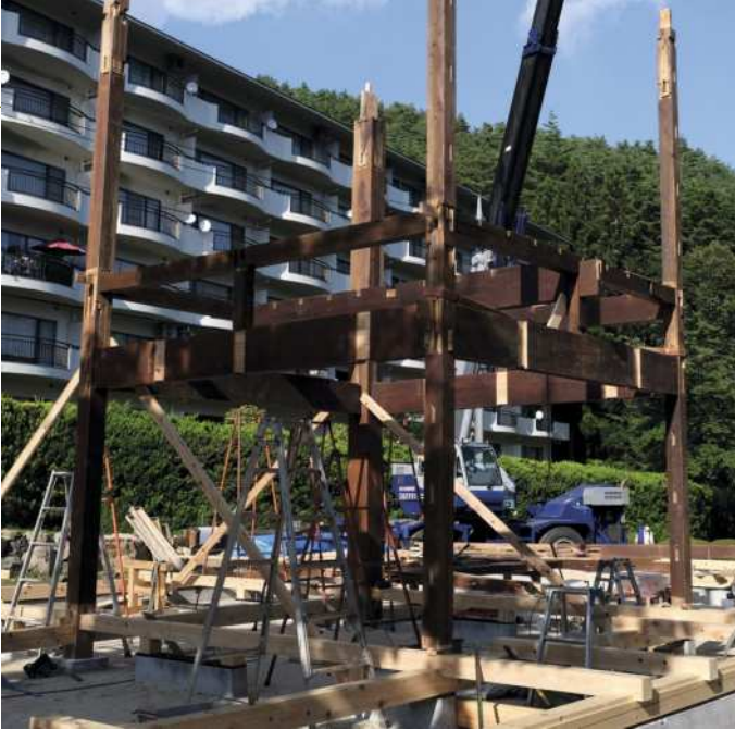
The first posts and beams standing (above). The long posts and the way the beams intersect did make for a technical assembly, requiring the posts to be slightly lifted and tilted to get all the beams in
