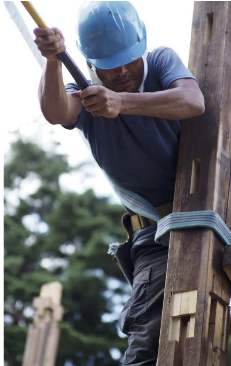
Naturally, we all settled into our roles, those who enjoy being up taking the reins and hammering the materials. Others were in charge of tying the materials, supporting the posts, making minor adjustments amongst others
