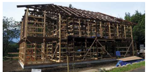
The signs of repair (left) are visible on the posts. Having stood for almost a century, it's inevitable to have damage from the natural elements. As much of the damage was on the surface, a little patch made it almost good as new. The completed assembly (above), with the materials all back into their original positions. Next is to work on the roof, walls and interior, hopefully ready next Spring
