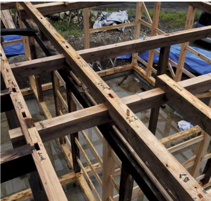
The second-floor beams I was in charge of. Repairing the old materials, working on the curved beams, marking and cutting out the new materials. This part is an extended area of the original structure
