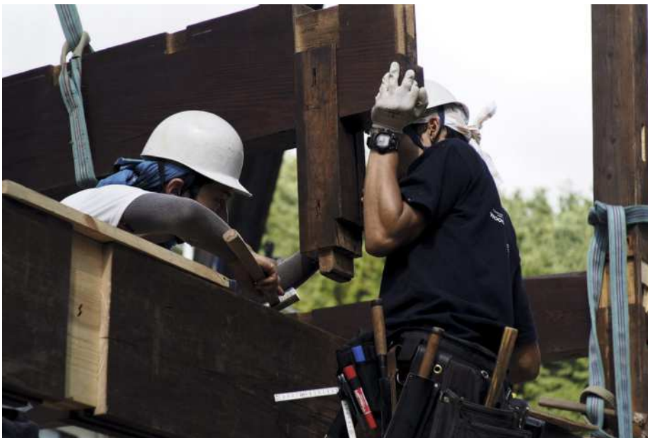
As not every joinery could be tested beforehand, some parts required minor adjustments on the go
