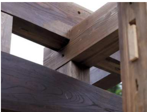
Curved beams, old and new materials, different heights, many things happening at once.
