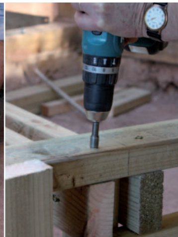
Check the spacer at the rear (above left) is square to the bed. Fixing the longest of the seat components to the back end of the bed (above)
