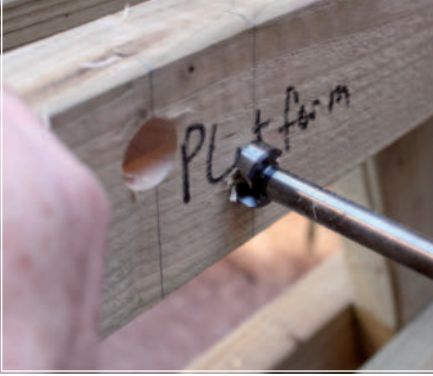
Drilling the platform with a Forstner bit (above) for the pivot, or use and auger (left)
