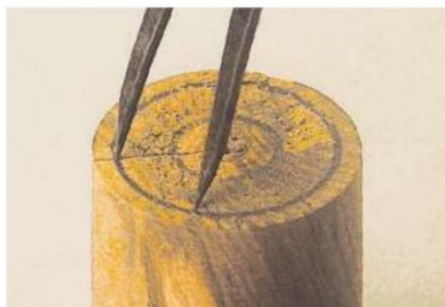
3. Alternatively, use dividers set 25mm apart to mark off six steps round the circumference
