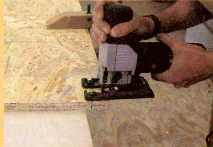
Cut both bottom panels to size; then clamp them together and cut 1 1/2in. notches at each corner.
