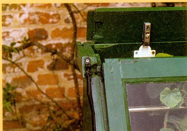
Fit a window stay. Cut out frame to accommodate peg.
