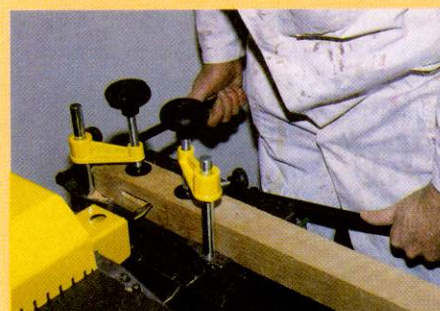
7. Typical mortising taking place.
