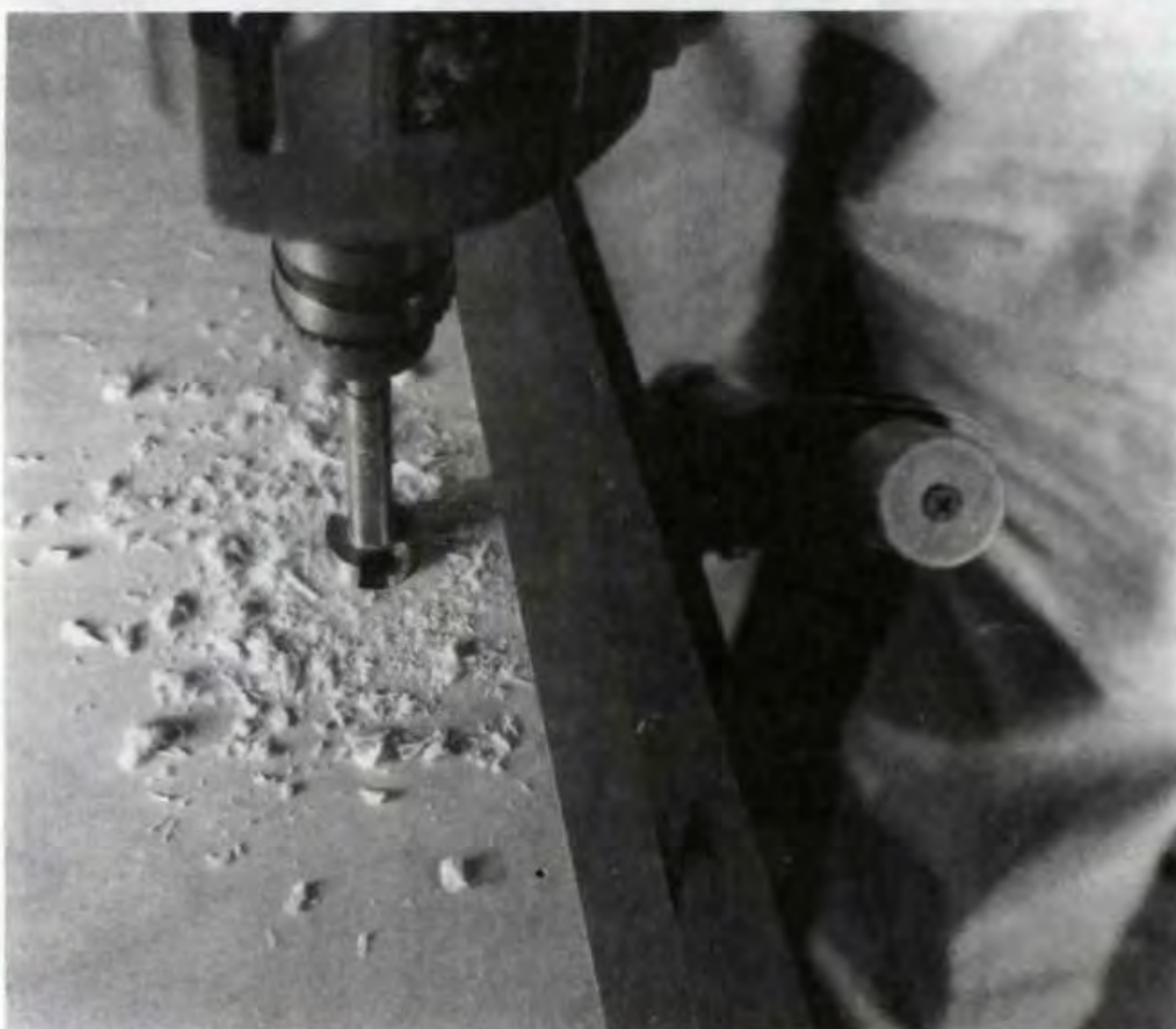
Figure 2. Use a backer board when drilling the hole into the door to prevent excessive wood splintering.
