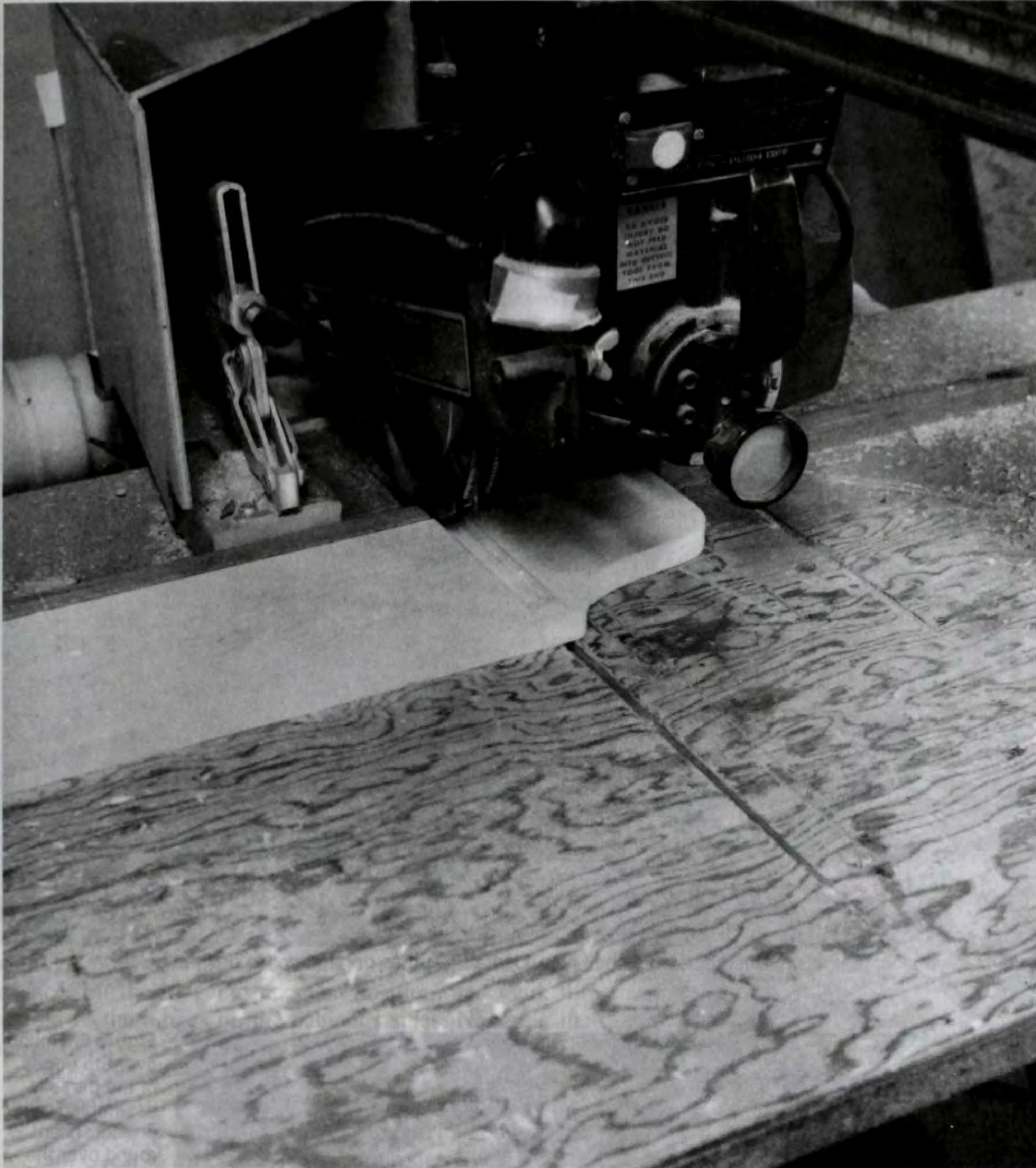
Figure 3. Cut a stopped dado for the top and bottom workpieces. Carefully mark the stopping points on your saw.
