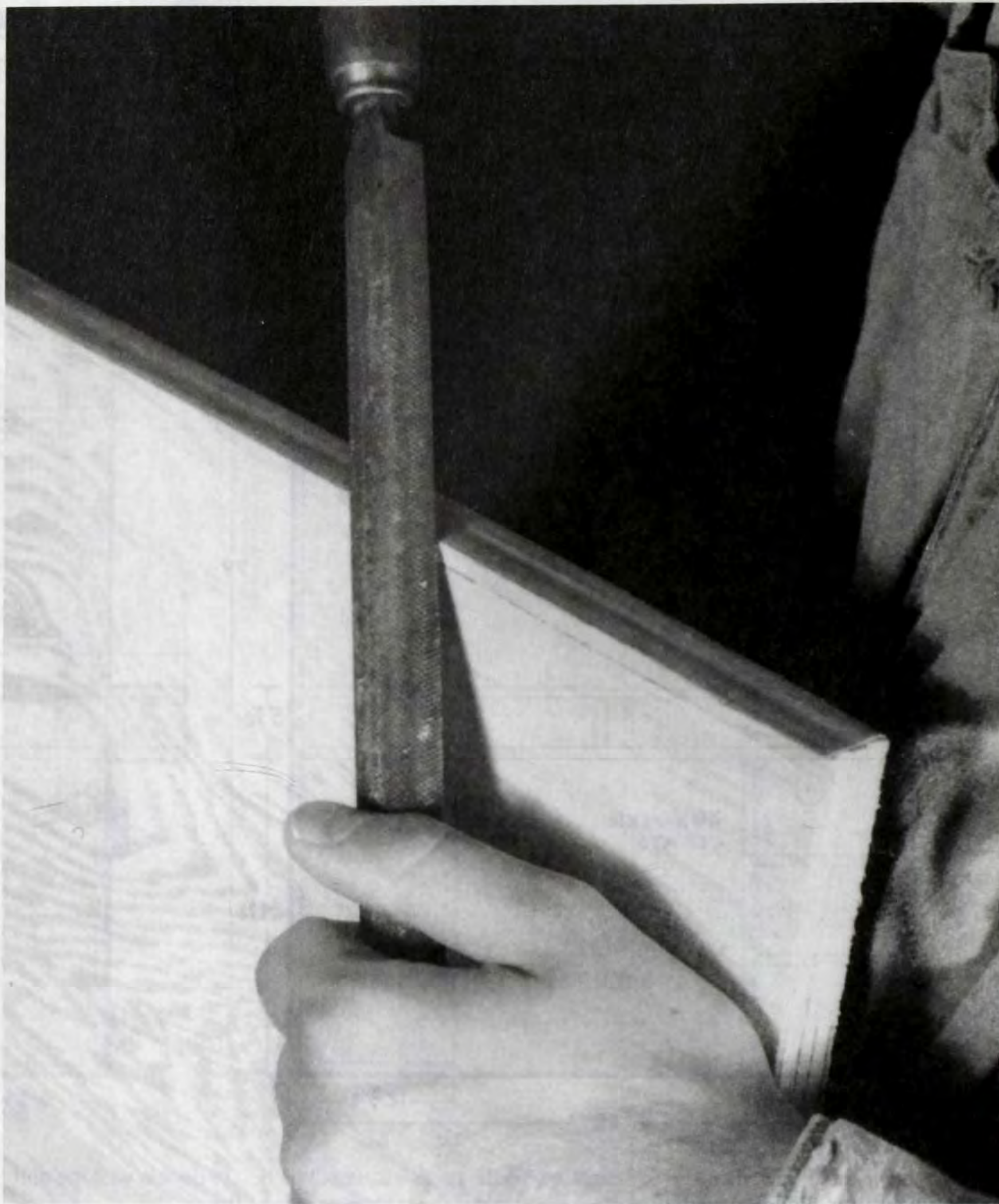
Figure 3. Remove excess edging by filing into the edge as you move the file forward. Work slowly. Then sand the edge to suit.
