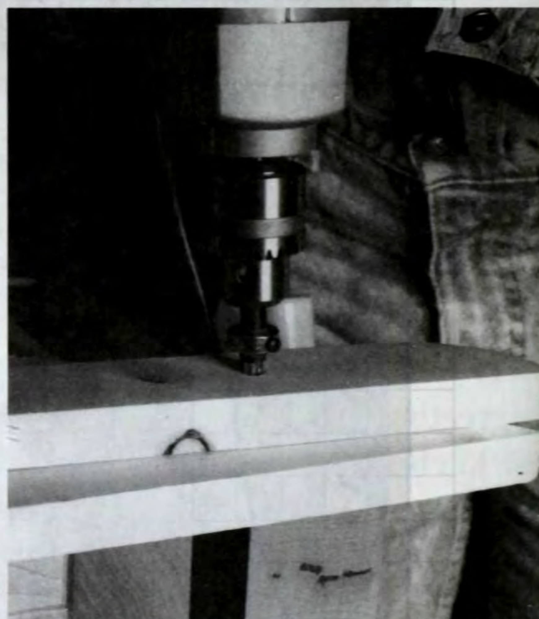
Figure 4. Here the holes for the screws are being pre-drilled and countersunk at the same time. One such handy tool is made by Stanley and called the Screw-Mate. It comes in a variety of sizes, suited to the fastener size used.
