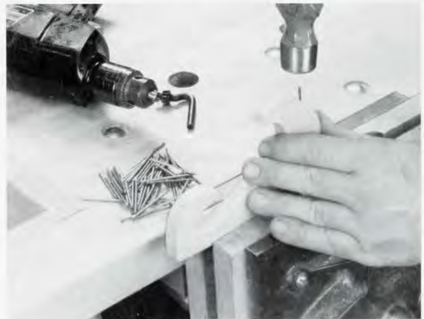
Figure 8. ...then remove the drill and hammer the nails home.
