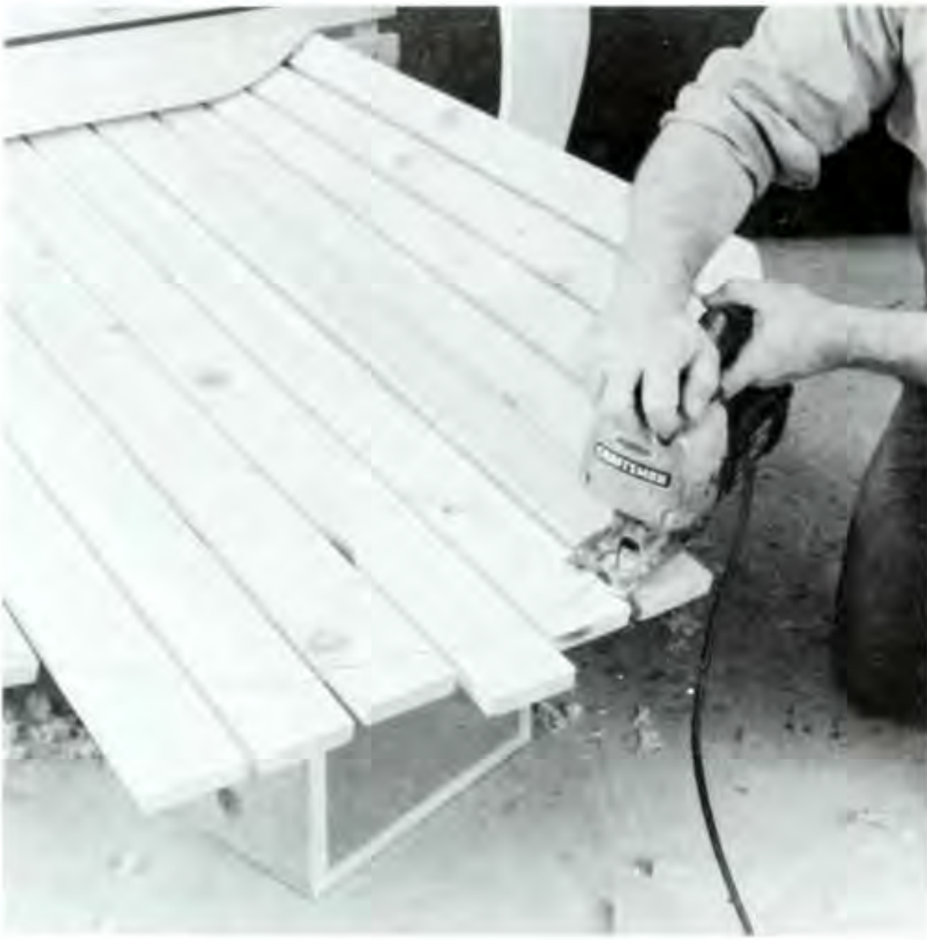
Figure 3. Cut the shape of the back with a sabre saw.
