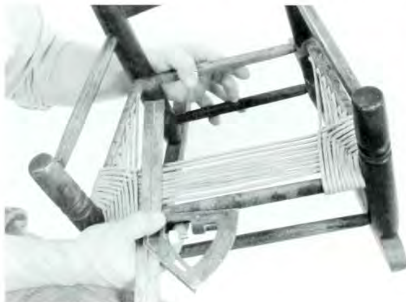
Figure 6. Every few rows, check your work with a combination square to make sure the warps and woofs are perpendicular.
