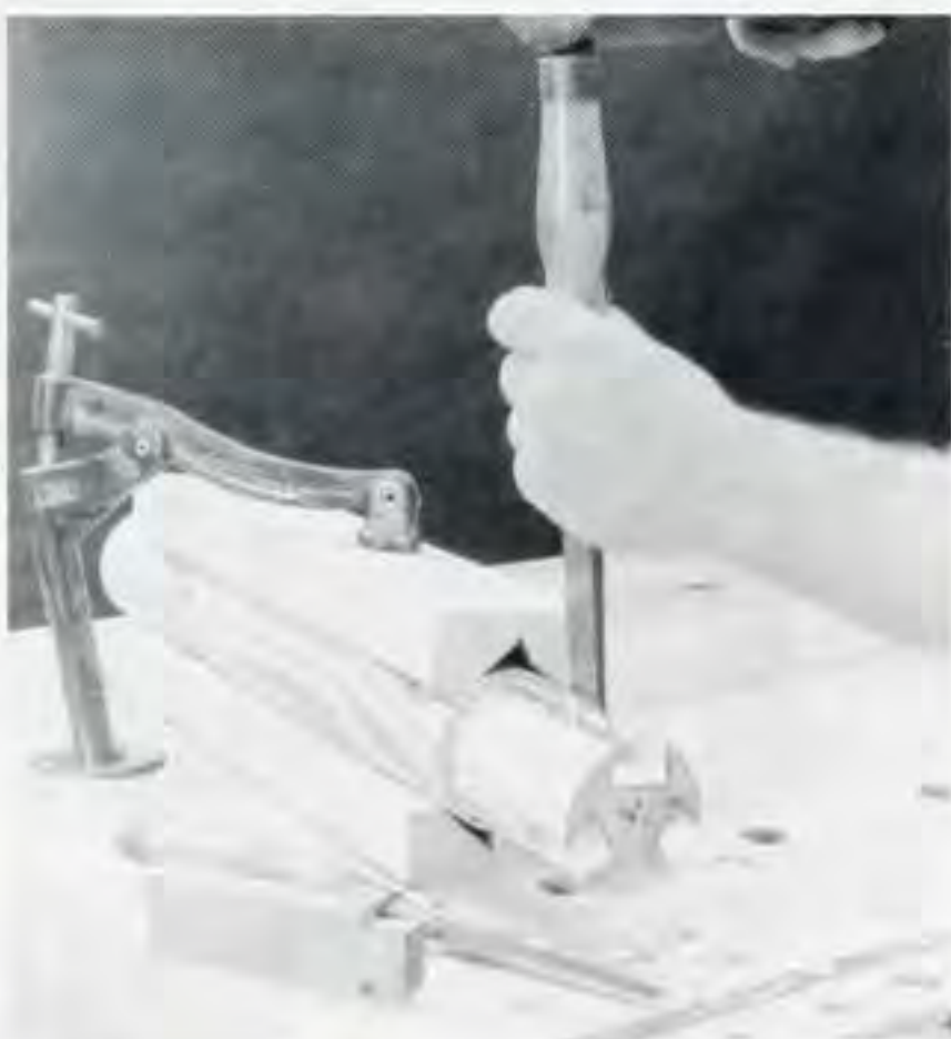
Figure 5. Shape the legs with a drawknife or a spokeshave, tapering them at the ankle so that the foot appears bulbous.
