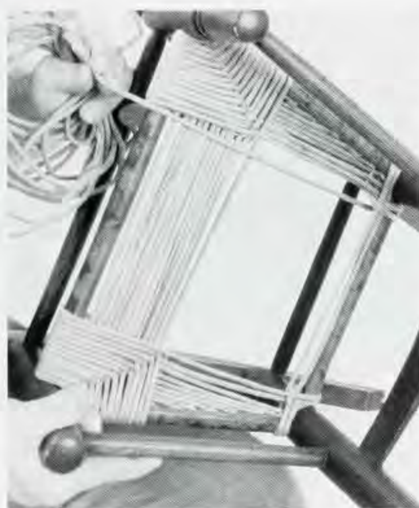
Figure 11. After you completely cover the side rails, begin a front-to-back weave to fill in the middle of the seat.
