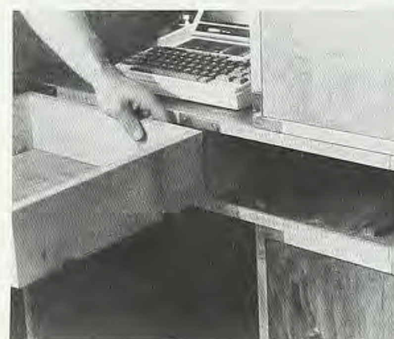
Figure 8. Full-extension drawers are mounted on extension slides. Notice that the front of the drawer is 'faced' with a piece of plywood.
