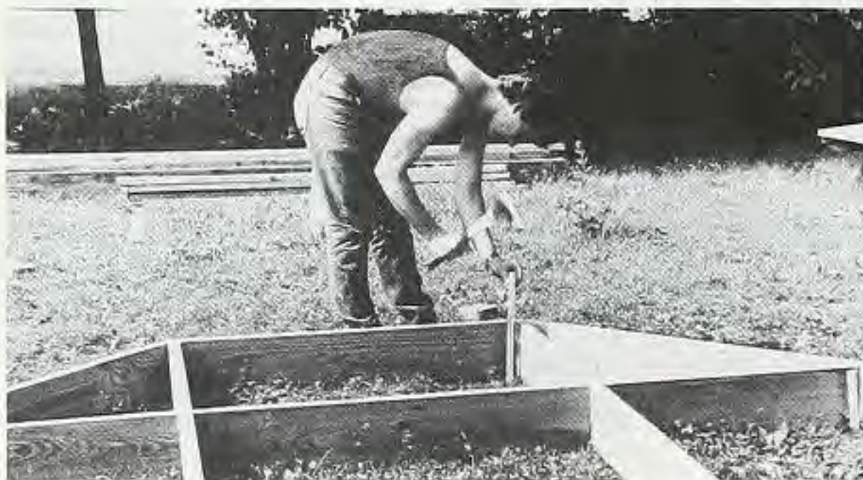
Figure 3. Put the floor frame in place on the building site, and mark where the posts will go with stakes.
