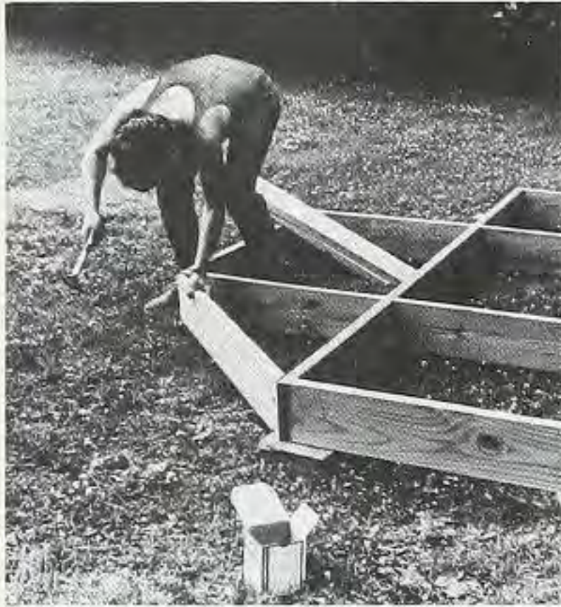
Figure 1. Assemble the 2 x 8 joists with lap joints. The joists will form a grid, like a tic-tac-toe game.
