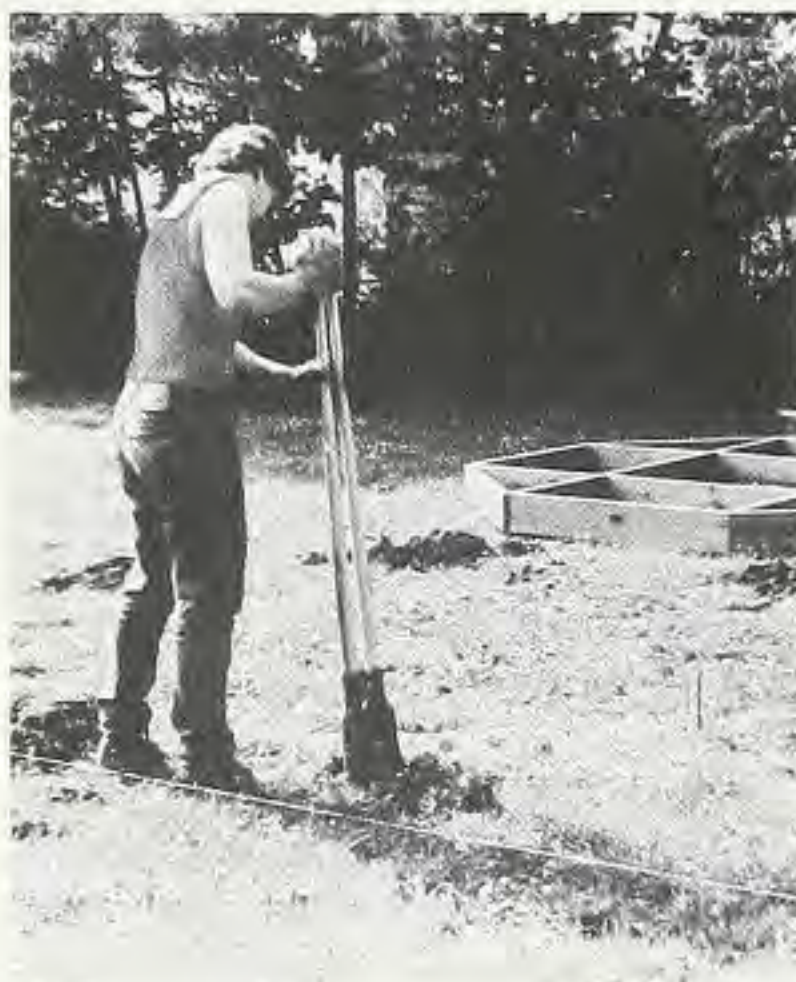
Figure 3. Put the floor frame in place on the building site, and mark where the posts will go with stakes.
