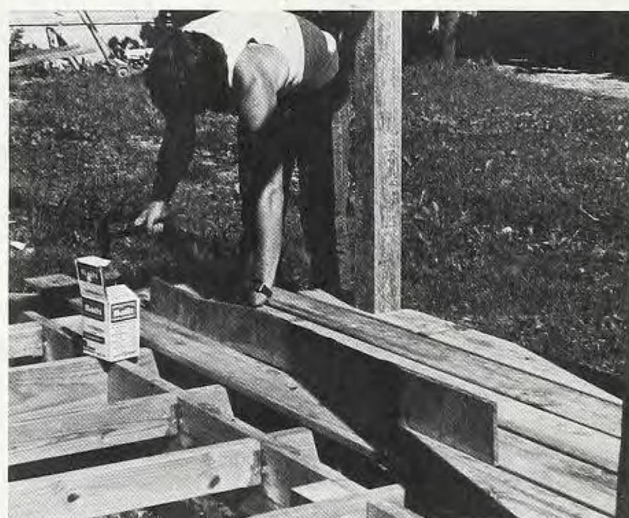
Figure 12. Install the decking with spiral nails, spacing the planks \frac{1}{4} "- \frac{1}{2} " apart. If you wish, use a thin board to get the spacing even.
