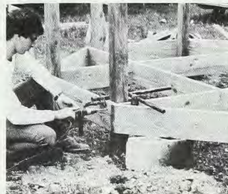
Figure 7. Attach the posts to the floor frame with lag screws.
