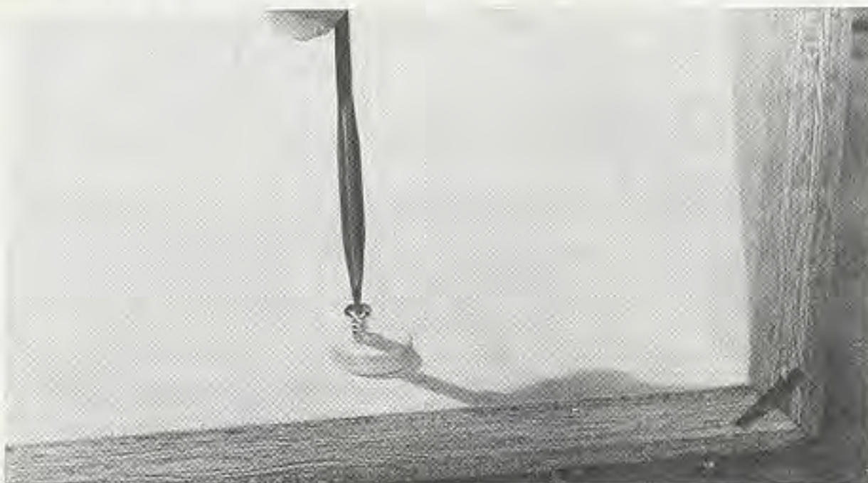
Figure 11. To make an adjustable door stop, cut a small wheel from \frac{1}{4} " plywood and drill an off-center pilot hole for the mounting screw. To adjust the stop, just turn the wheel.
