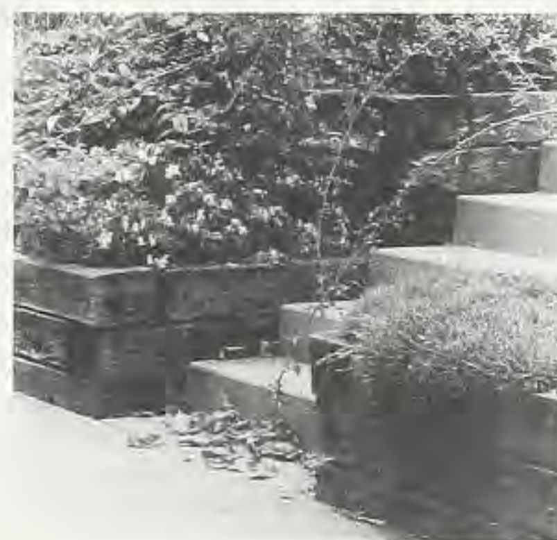
Figure 1. Railroad ties and creosote-treated lumber should be used for garden landscaping only after it's weathered for many years. Newly creosoted timbers may be harmful to plants.
