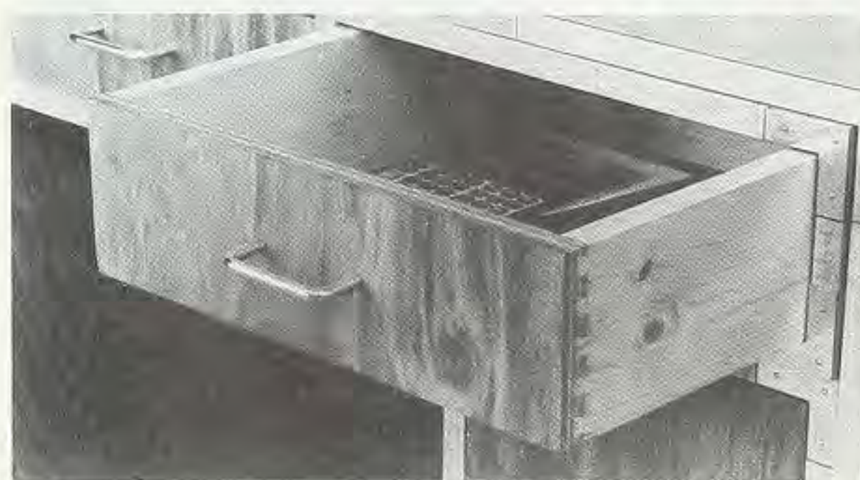
Figure 7. Plain drawers work best in the smaller boxes — those that are either 5\frac{7}{8} " or 11\frac{3}{4} " high.
