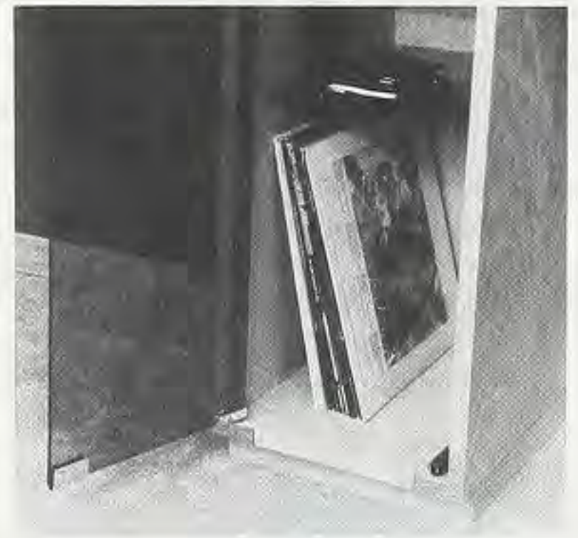
Figure 13. Drop-leaf doors are mounted on special drop-leaf hinges. Drop-leaf supports help to keep the doors horizontal, even when used as a shelf or desk.
