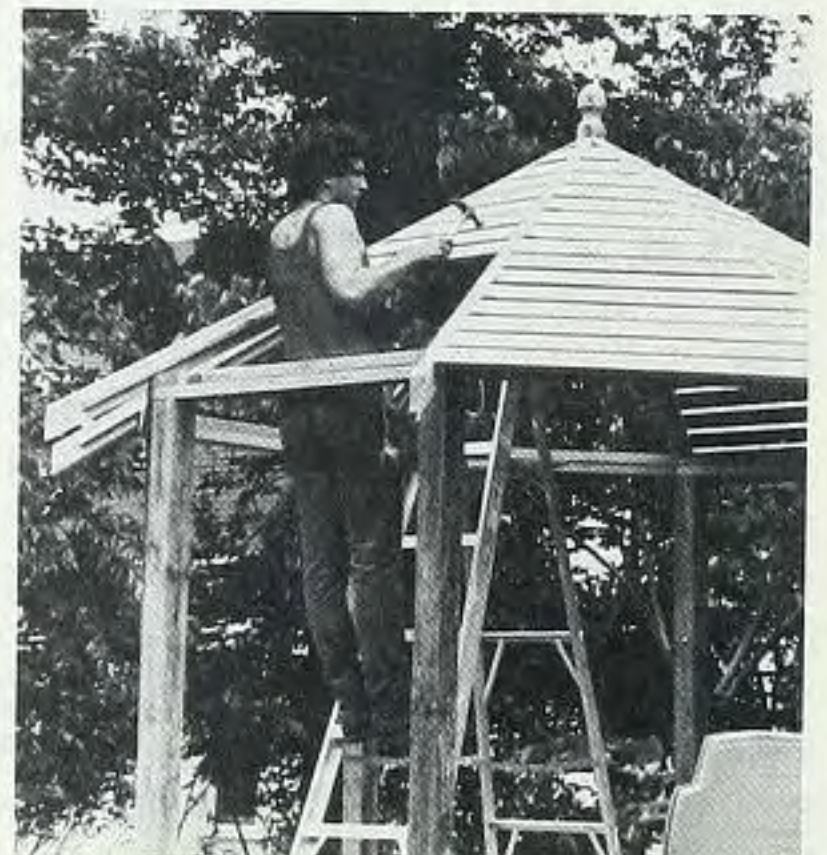
Figure 14. Hand fit the roof slats, compound-mitering the ends. Nail them to the cleats, beginning at the top of each section and working your way down.
