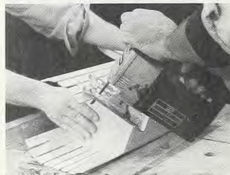
Figure 5. After the glue has dried for several hours, cut the wing strip to the proper length and angle with a saber saw. Have a helper hold the assembly while you cut.
