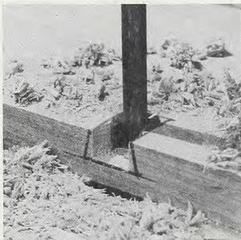
Figure 6. Then remove the rest of the waste with a hand chisel.
