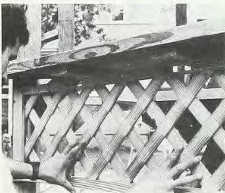
Figure 17. Notch the lower frames so they fit around the battens on the undersides of the seats and shelves.
