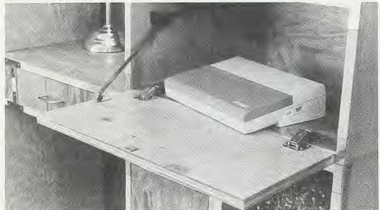
Figure 13. Drop-leaf doors are mounted on special drop-leaf hinges. Drop-leaf supports help to keep the doors horizontal, even when used as a shelf or desk.
