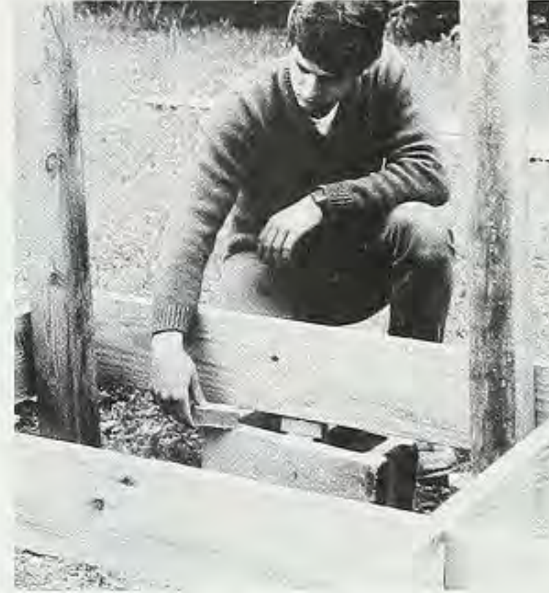
Figure 2. Nail the floor frame members to the outer ends of the joists to make an octagon. Attach the members with square-cut ends first, then the members with mitered ends.
