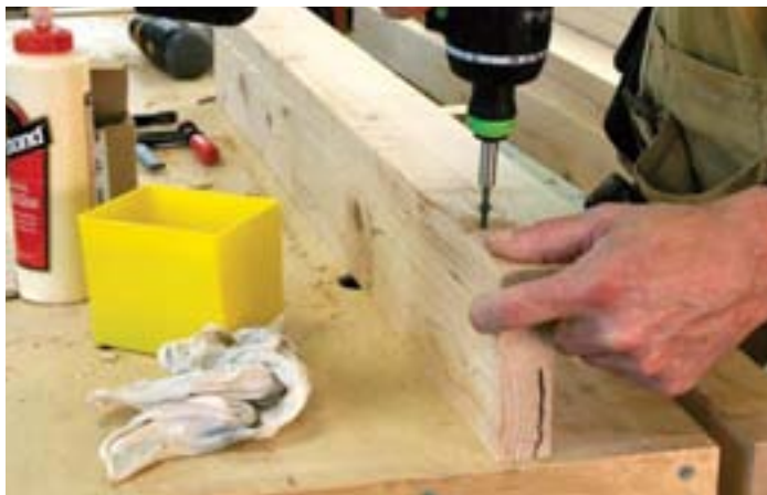
All together now. With the frames inside the leg assemblies, this table is ready for a plywood shelf and top.
