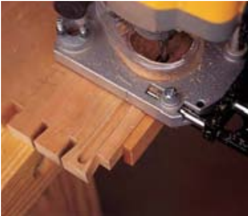
On the tail boards, you need to stop the groove in one of the tails as shown. The dovetail layout shown in the illustration allows you to put the groove solidly into a tail.
