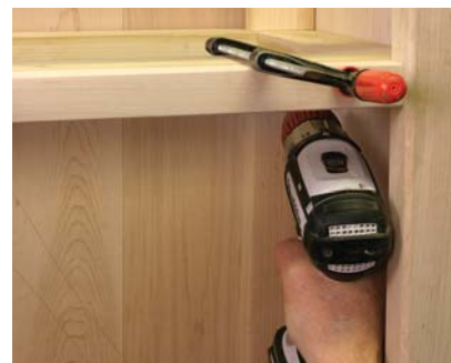
A pocket screw at each end attaches the drawer frame to the inside of the back legs.
