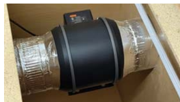
RIGHT Once the exhausts are joined, the ductwork expands to 6" and exhaust is pulled out of the workshop by this powerful 6" inline fan.
