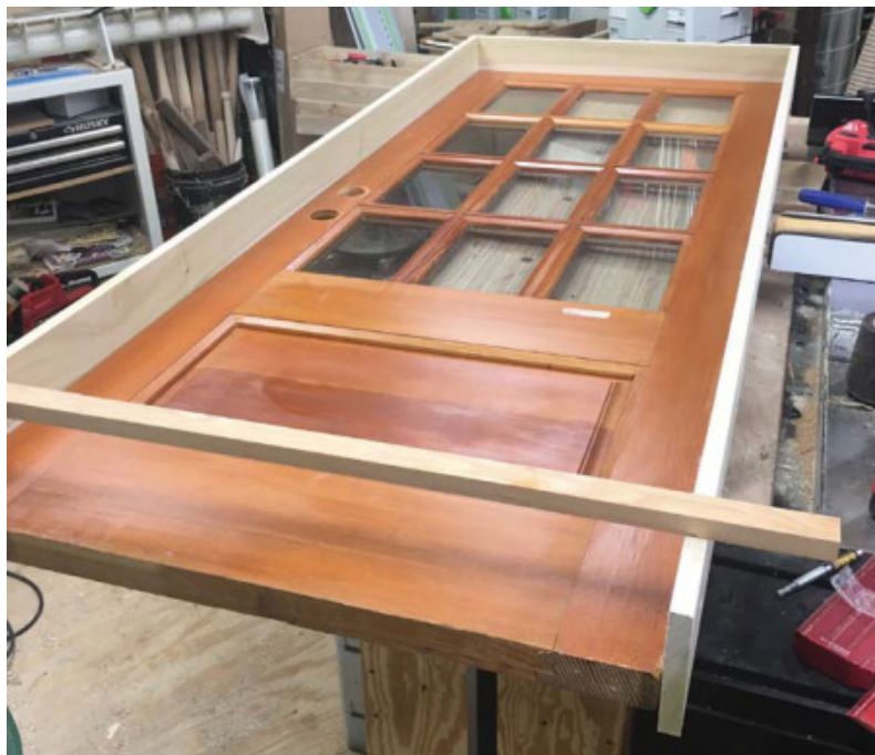
The kitchen door. Made mostly of Douglas fir (I think), with a cherry-ish stain. A little trimming of the door, a shop-made jamb, some new hardware, and it fit right into the kitchen, even though it's not what we'd originally planned.
