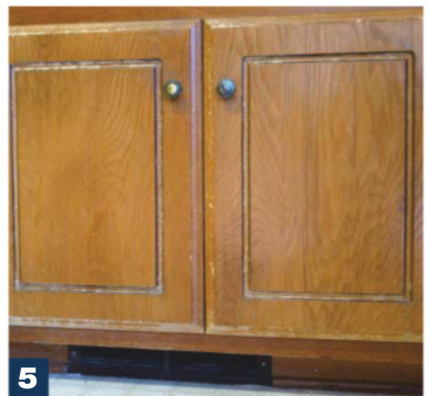
5 A common problem when finishing cabinet doors is not getting a thick enough finish on the edges. Especially under sinks, this can result in the finish peeling long before it should.
