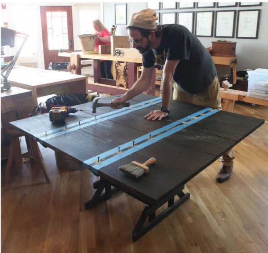
Finish nails. Nails move with the seasons and, when properly installed, hold quite well. Also, I think modern screw heads are ugly. The blue tape helps guide my drilling.
