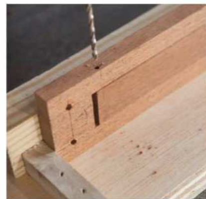
Make a hinge. Drill a \frac{3}{32} " hole through the middle assembly and kickstand. Then use a nail as the barrel of the hinge.
