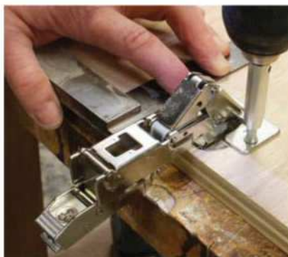
Square up. Use a square to position the hinge while drilling with a Vix bit.
