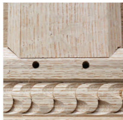
All together now. One of the chest's joints during a test fit. This is as good as it needs to be.
