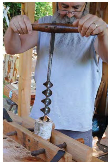
Boring bit. Use a 2"-diameter auger bit to remove the bulk of the interior waste.
