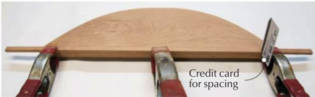
Less conspicuous. By gluing in place the last inch or so on each end of the wall half of the cleat, it will help hide the cleat when viewed from the side once the piece is on the wall. (In this picture, the ends still need to be flush cut to the shelf's curve.)
