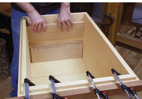
This high. The 5 1/4"-wide spacer acts as a shelf when installing the runner above it. The 5 1/4" height is critical for holding standard bench planes below the bottom tray.
