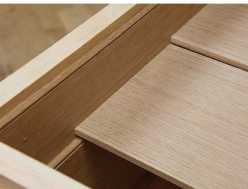
Smooth-sliding bottom. The bottom boards are the only part that touches the runners. So shoot them to perfect length until you get the sliding action you want with zero racking.
