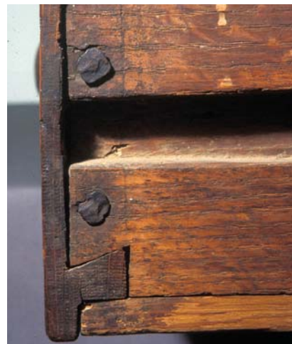
Nailed tails. While they are rare, there are a few surviving examples of 17th-century dovetails. But most feature nails through the tail board.
