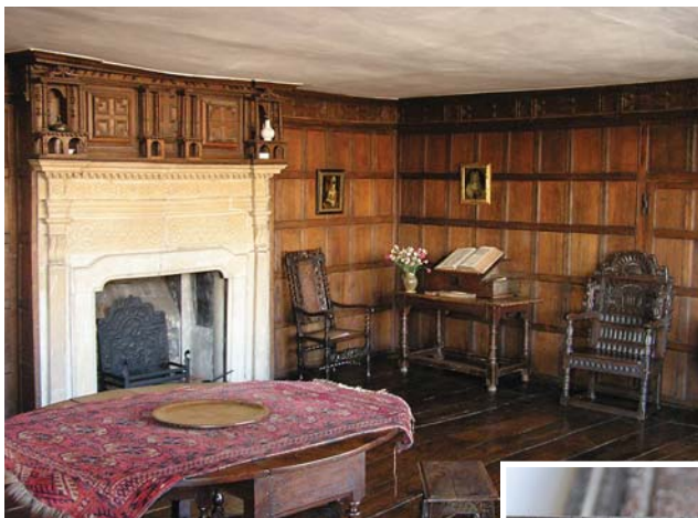
Wainscot. The hall in the Merchant's House (Marlborough, Wiltshire) shows period wainscoting; a room or two like this could easily use "half a hundred" muntins. The inset photo (below) shows a cross-section of a wainscot muntin (notice the drawbore holes).
