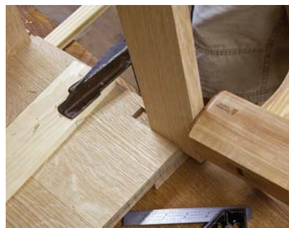
Knock & nail. Drive the interior rail in place. Then fasten it from the outside of the case with two 6d rosehead nails at each end.
