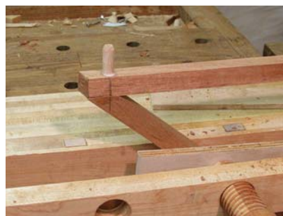
Stopped hole. The cross braces are securely attached to the side stretchers using 3/8" dowels. Take care not to drill all the way through the show face of the cross-brace pieces.
