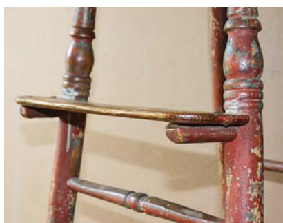
Afterthought. Most footrests on Windsor high chairs are later additions, often poorly executed.
