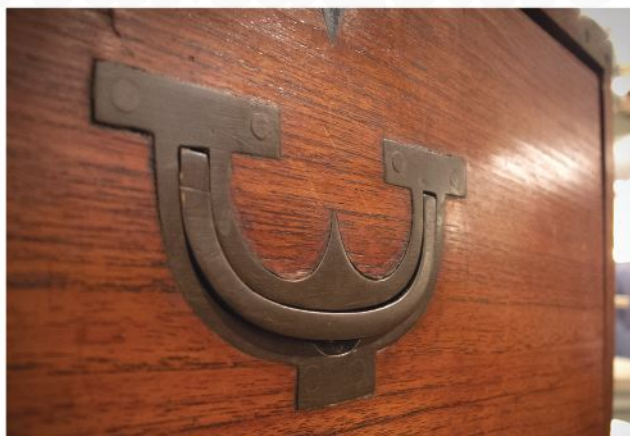
A 'rivet.' This piece of early campaign hardware is held in with screws that then had their heads filed off flush to the pull. This feature shows up on other pieces and even on English handplanes.
