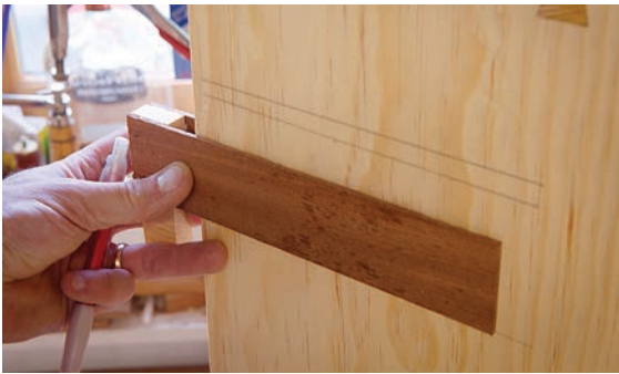
Affix the dividers. With the lines drawn on the carcass sides, drive in the cut headless brads and set them 1/16" below the surface.
