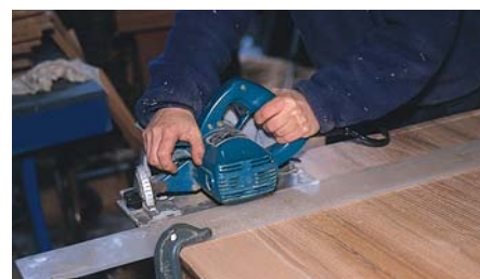
It takes two. To trim the end of the top, the circular saw blade was too small to cut through the entire thickness. The cut was completed with a kataba Anahiki-Nokogiri, a Japanese saw.
