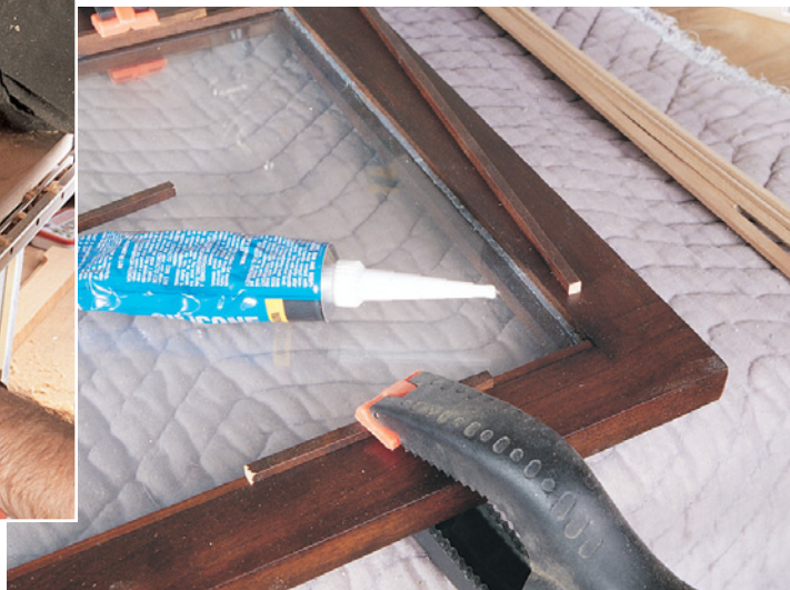
Put down a thin bead of silicone in the rabbet, then put the glass on that. Then lay down another bead of silicone and press the wooden retaining strip into place to cover the goop. Now your doors look good when both open and shut.
