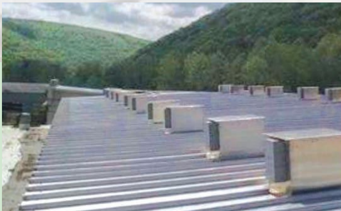
▲ Kiln roof replacements
