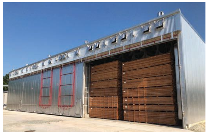
Y&Y Hardwoods in Thomasville, NC has four Package Kilns.
