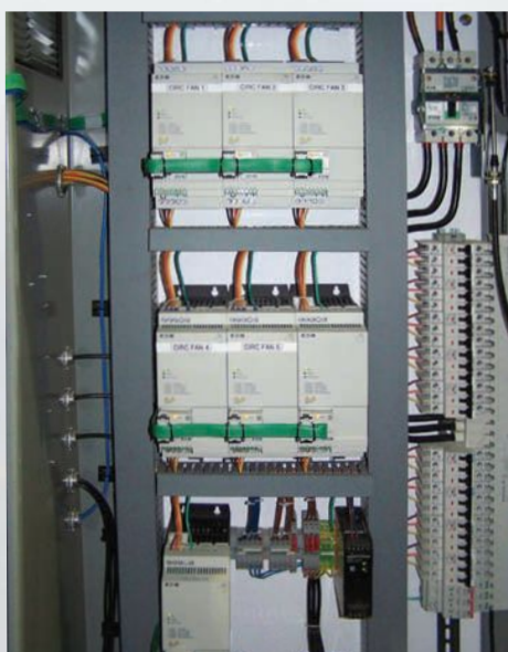
◀ Individual drives for circulation fan motors
