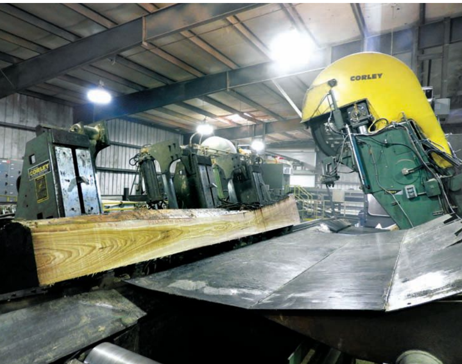
Cardin Forest Products operates a turn-key sawmill built by Corley Manufacturing featuring two 7-foot band mills where logs are made into cants, which are then processed by the 7-foot vertical resaw into grade lumber.
