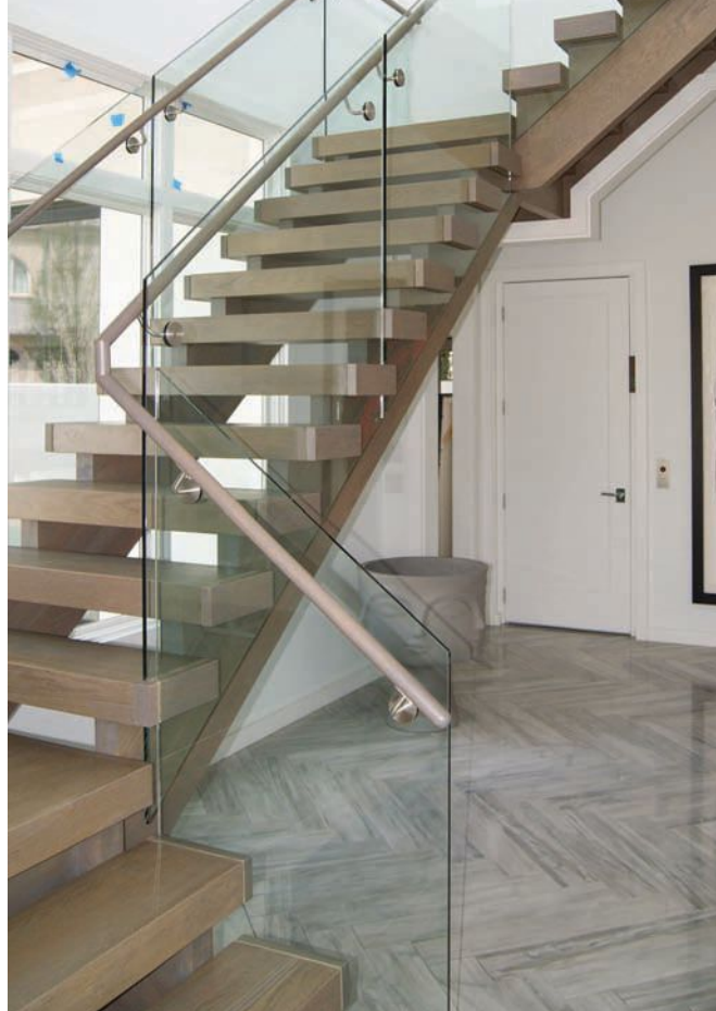
This is a freestanding stairway with open riser, cut stringer and an all-White Oak stairway. It includes glass panels and modern round White Oak rail.
