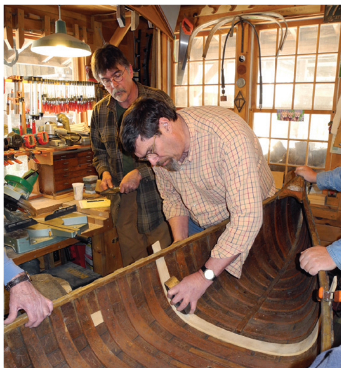
Clinching in new rib
