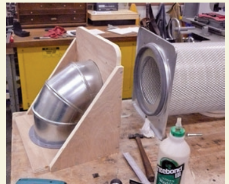
10—Transfer holes from flange to wooden support bracket
