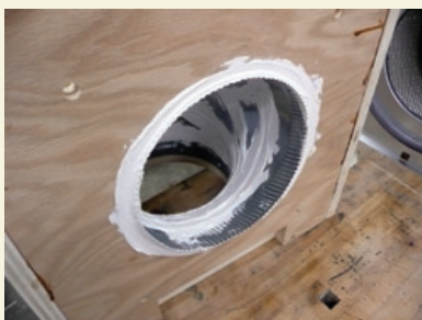
12—Sealing inside of 8" elbow with polyurethane caulk
