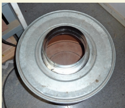
21—Installing flange on top of dust barrel
