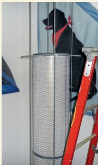
15—Assembly of filters to support bracket
