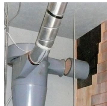
3—The sound dampener fitted thru the wall
