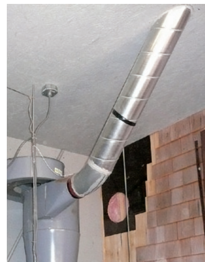
2—The cyclone disassembled, showing the start of the hole thru the wall
