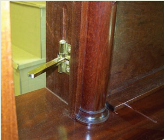
"Temple" hardware — temple is my term for box unit holding painted panels within the carved elements
