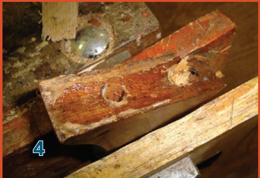
4 The joints were "coaxed" apart. A couple of the dowels were fractured in the process but were drilled out and replaced.
