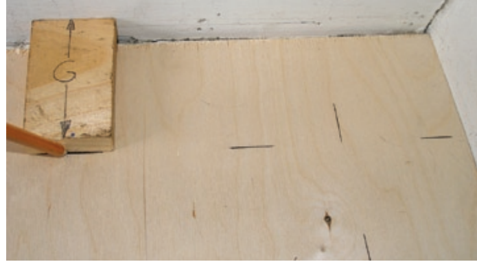
Photo #5 — Use of a gauge block
