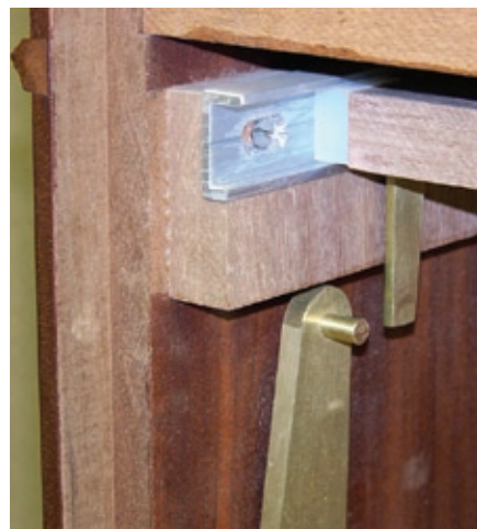
Detail showing lid/writing slide mechanism.
