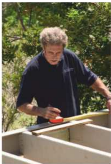
The spacing between the joists was measured to fit the blocking.
