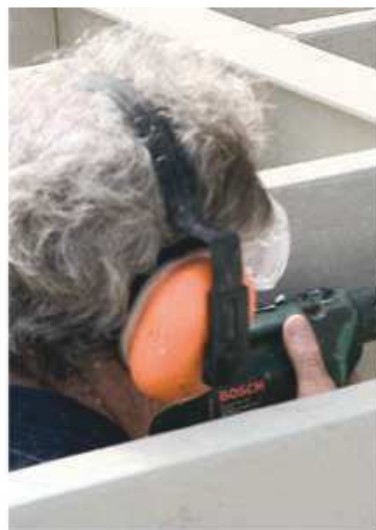
Clearance holes 5mm in diameter were drilled through the steel web.
