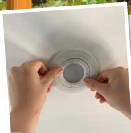
1 TWIST the downlight in an anticlockwise direction.
