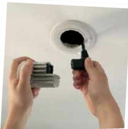
3 UNPLUG the downlight IEC plug and replace it with the new LED.
