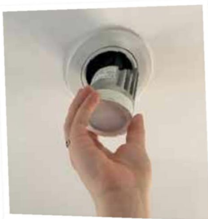
2 ALLOW the downlight to drop out and into your hand.
