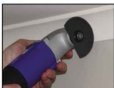
CUTTING PLASTER & CORNICE
