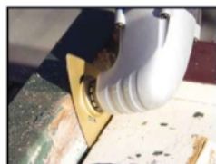
AGGRESSIVE PAINT REMOVAL
