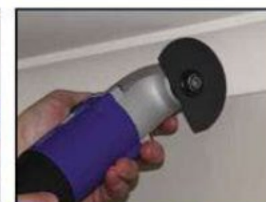
CUTTING PLASTER & CORNICE
