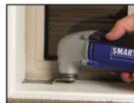
UNDER CUTTING DOOR JAMBS
