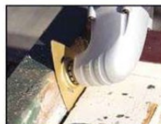
AGGRESSIVE PAINT REMOVAL
