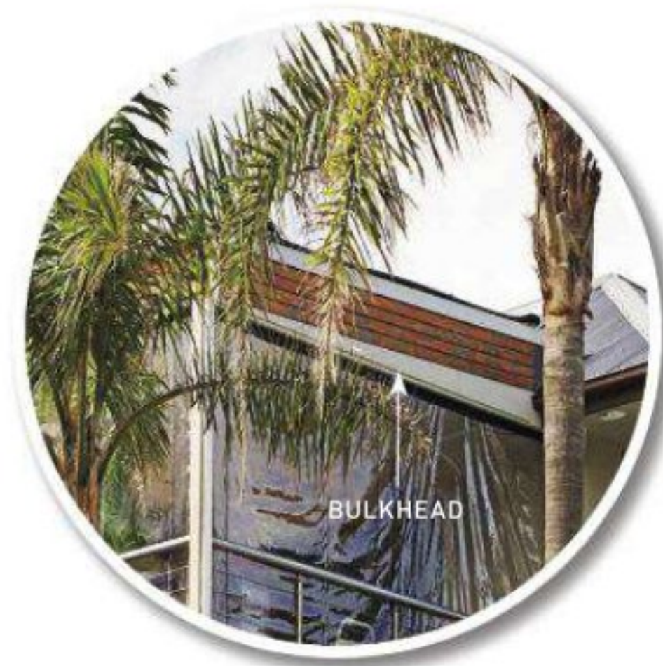
A triangular bulkhead allows head rails to be attached level under sloping beams.
