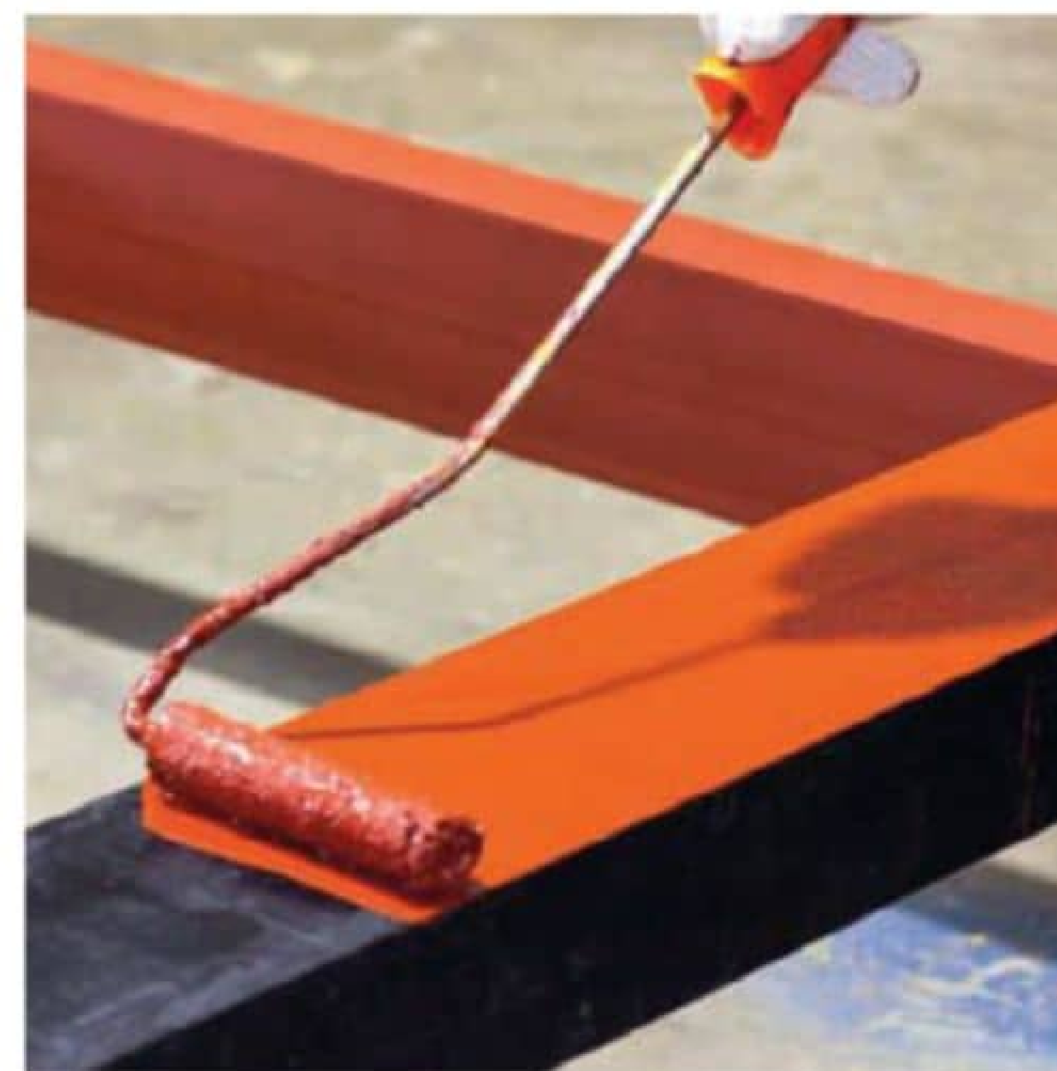
Before painting, clean the entire gate thoroughly
