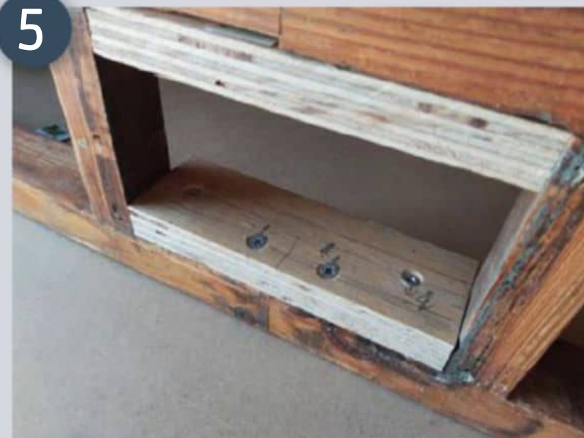
Screws driven at an angle
