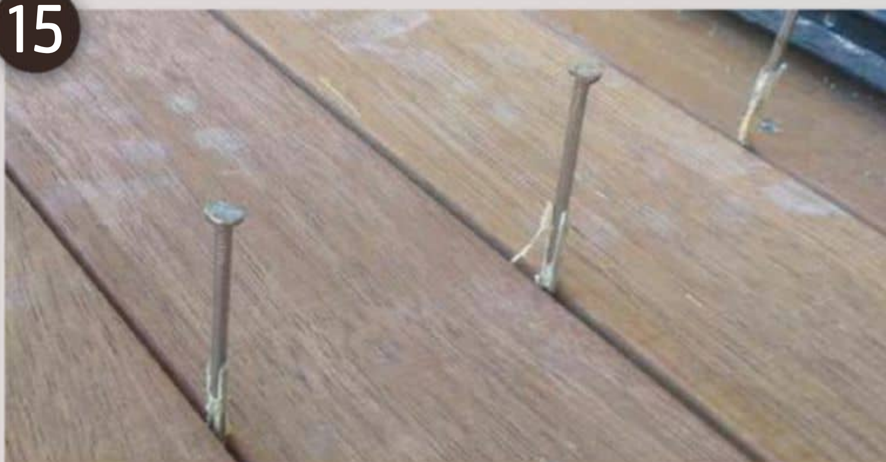
Timber decking needs to have a 3-4mm gap to allow it the expand
