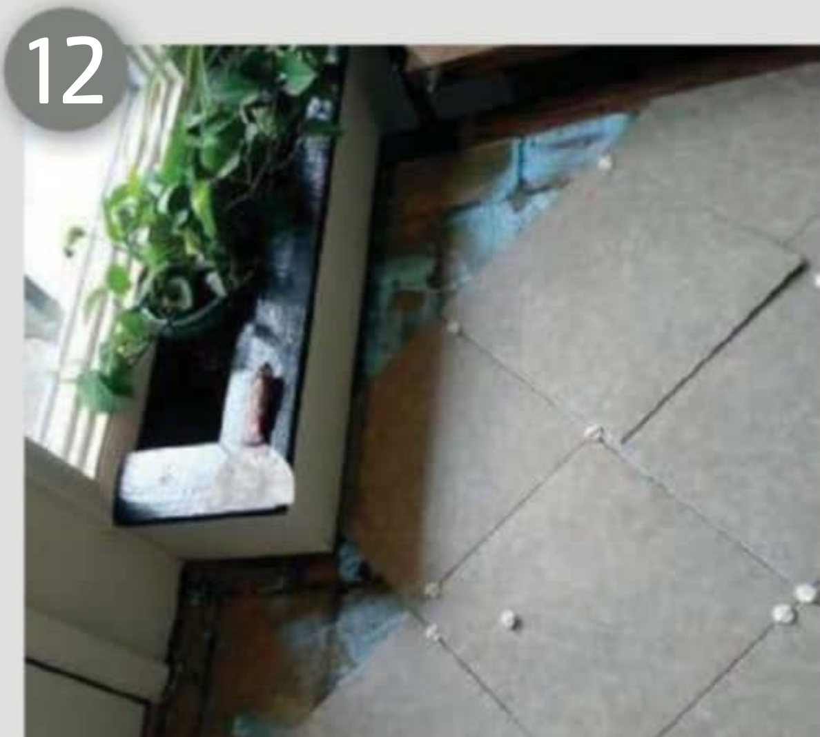
Measure and cut tiles to fit in the corners
