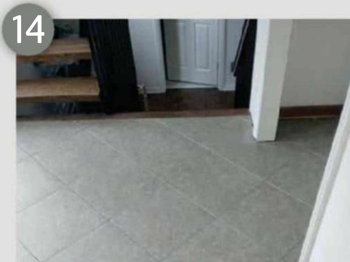
Once everything is set in place, pull the spacers and use your roller to apply even pressure all over the floor
