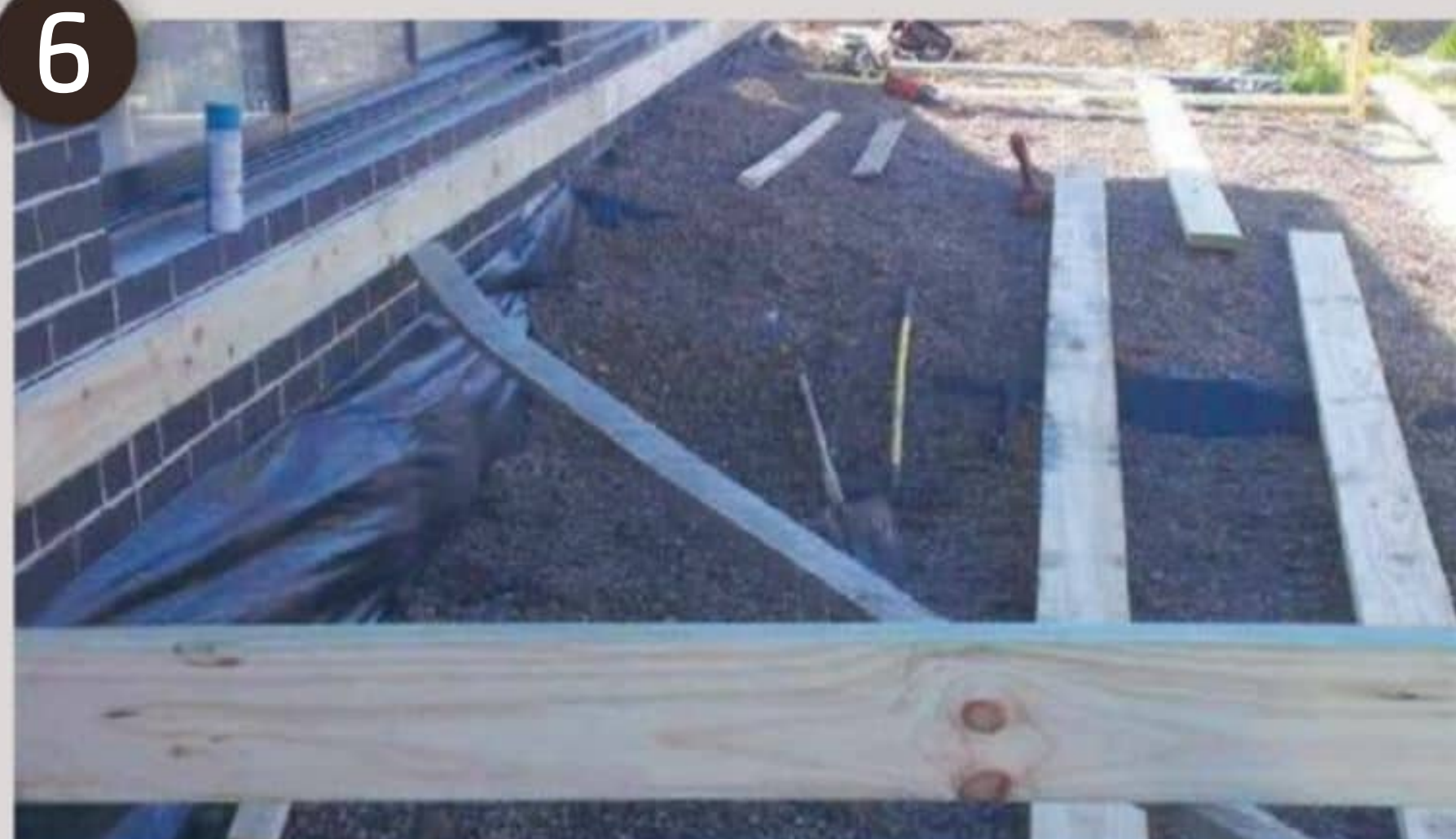
Make sure that your joist is perpendicular to the plate
