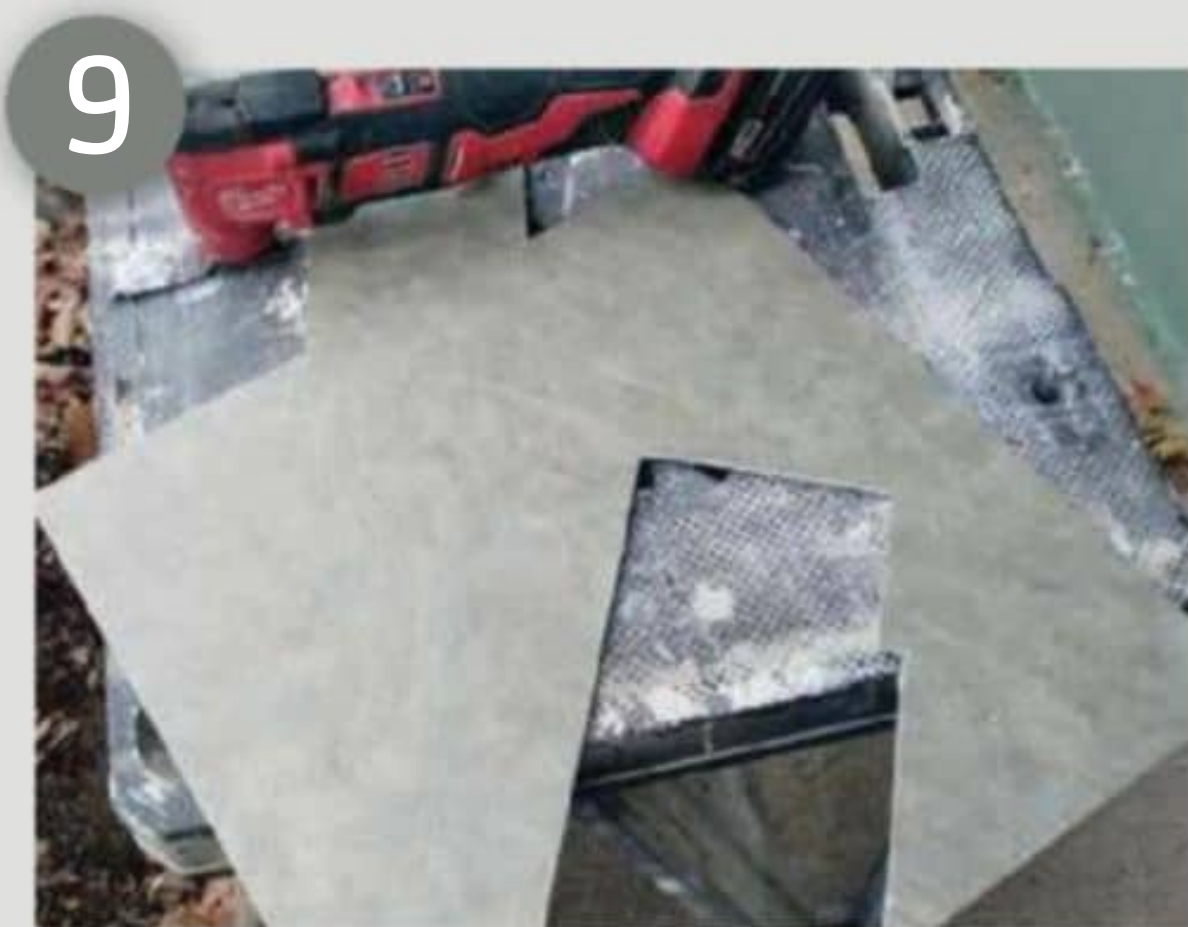
Measure, mark and cut the tiles
