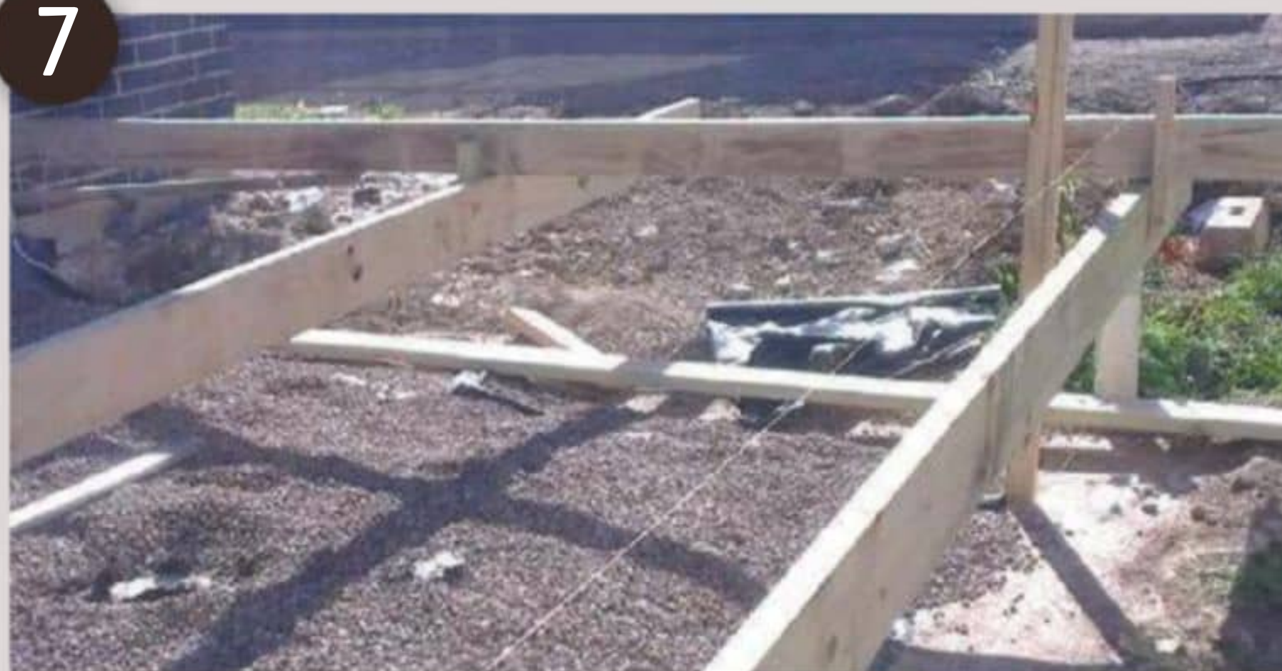
Use a string to run along the top of the joist from one end to another
