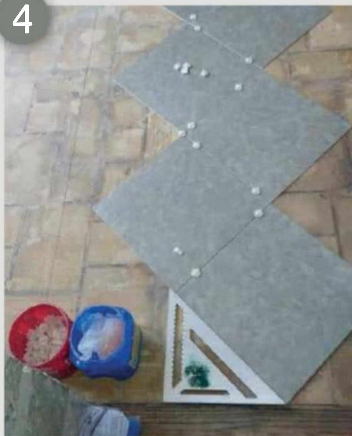
I decided to install this floor with a diagonal pattern
