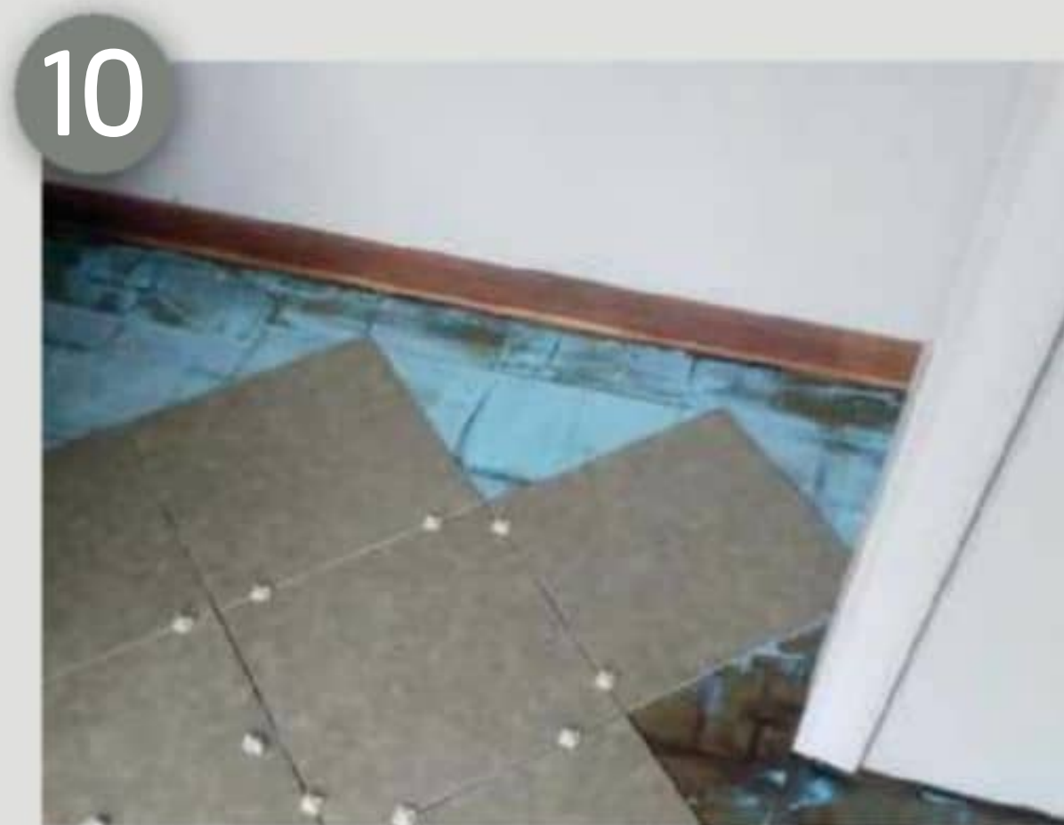
This was where the tile needed to go
