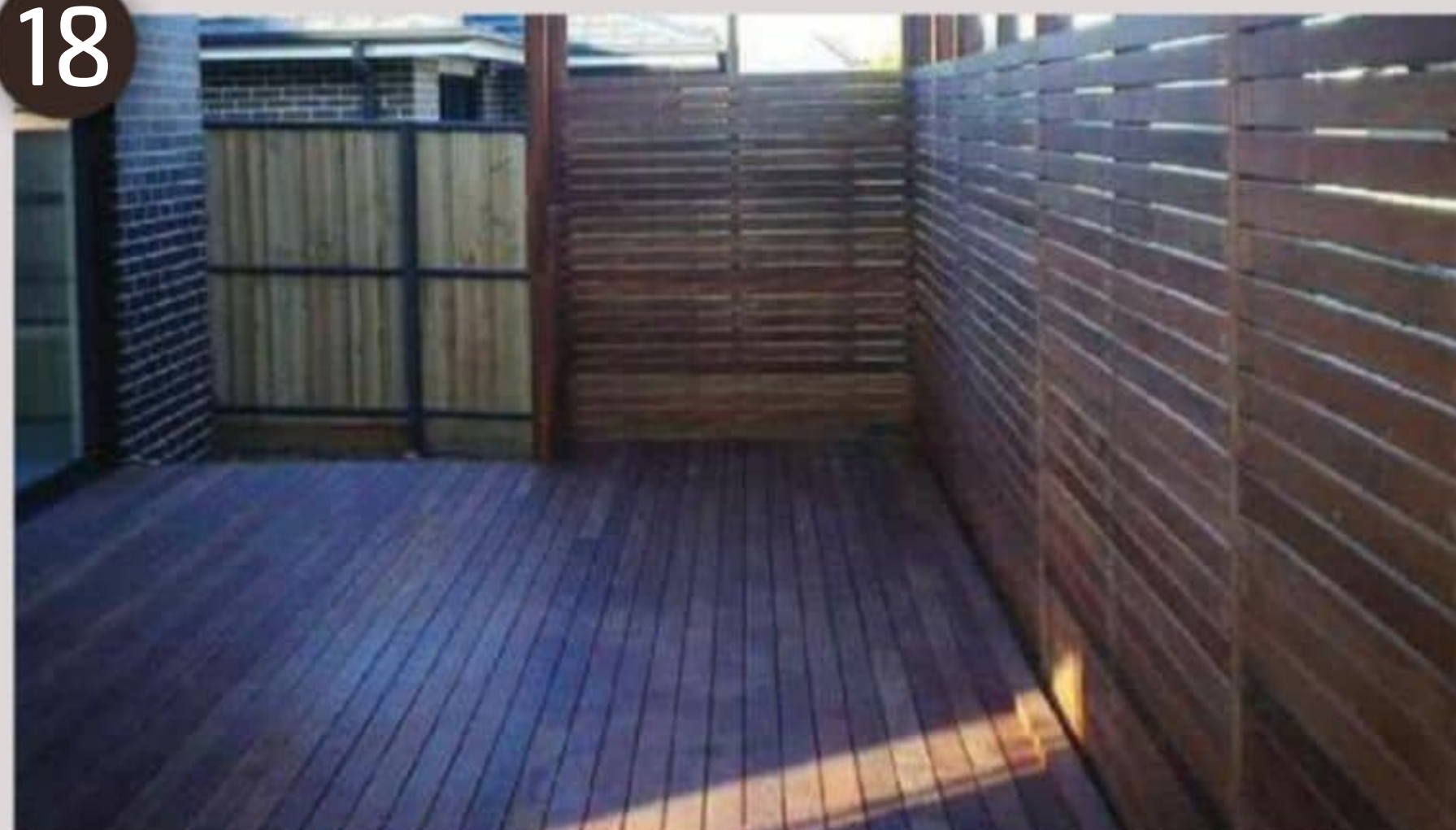
The deck all done
