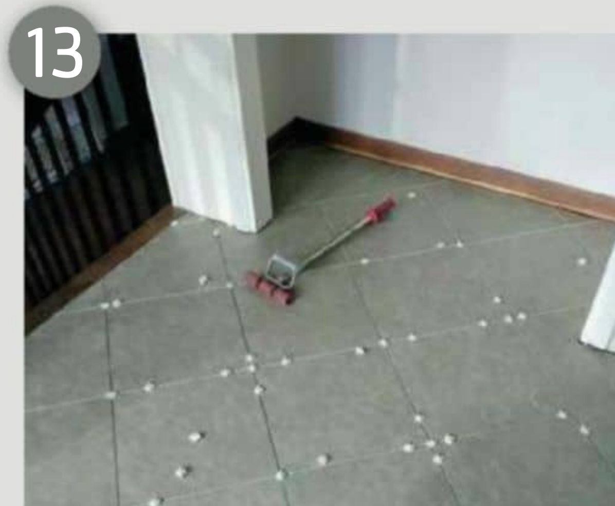
Use the plastic spacers to keep your grout lines even
