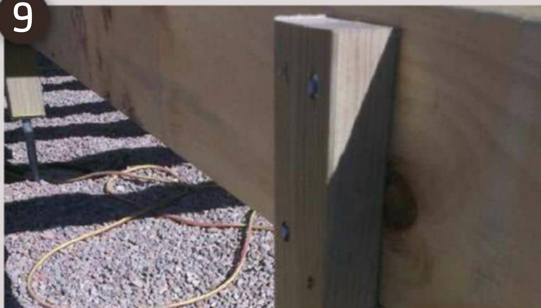
Nail or screw the bearers to the underside of the joist
