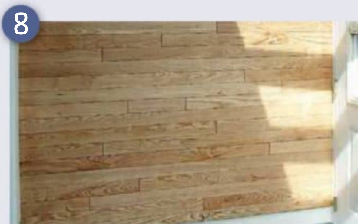
1. The pile of leftover hardwood flooring 2. The wood once it had been prepared 3. The wall in need of a feature 4. Start installing the panels from the bottom 5. Work your wall up the wall 6. All panels installed 7. Applying the finish 8. The wall once it had been varnished 9. If you have leftovers, find another wall to renovate
