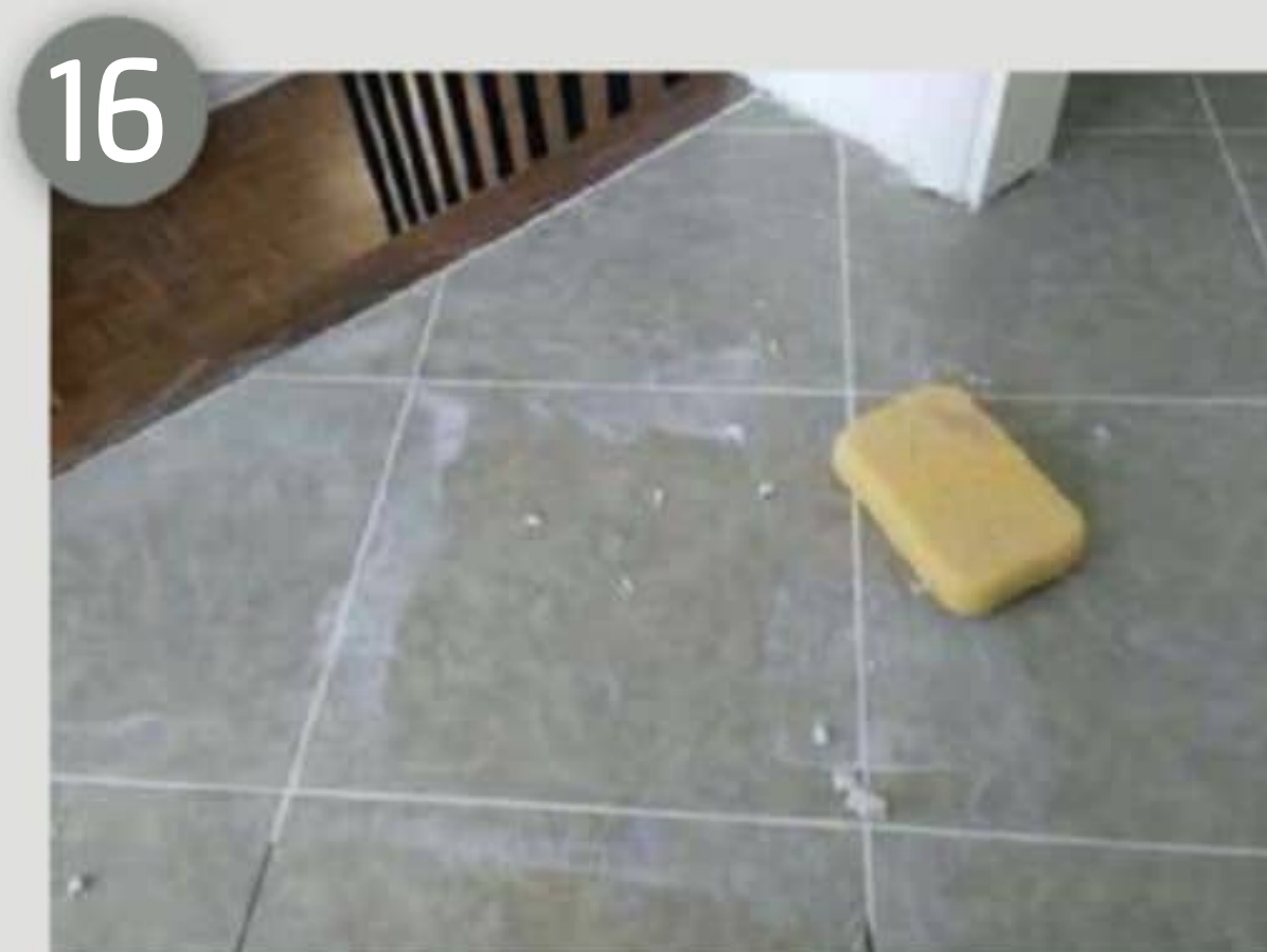
Apply grout to the joints, dress the lines with a damp sponge, then do a final clean-up with the sponge
