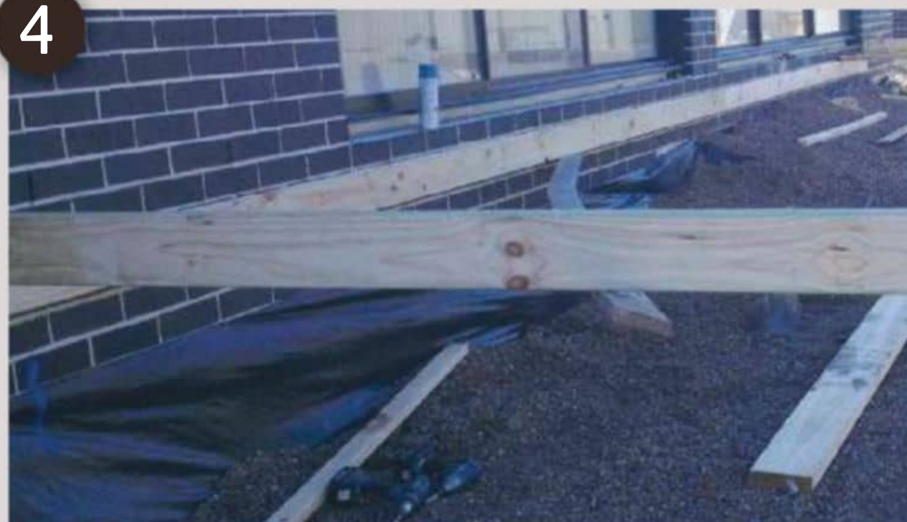
Set up the end joist, by nailing or screwing it to the plate
