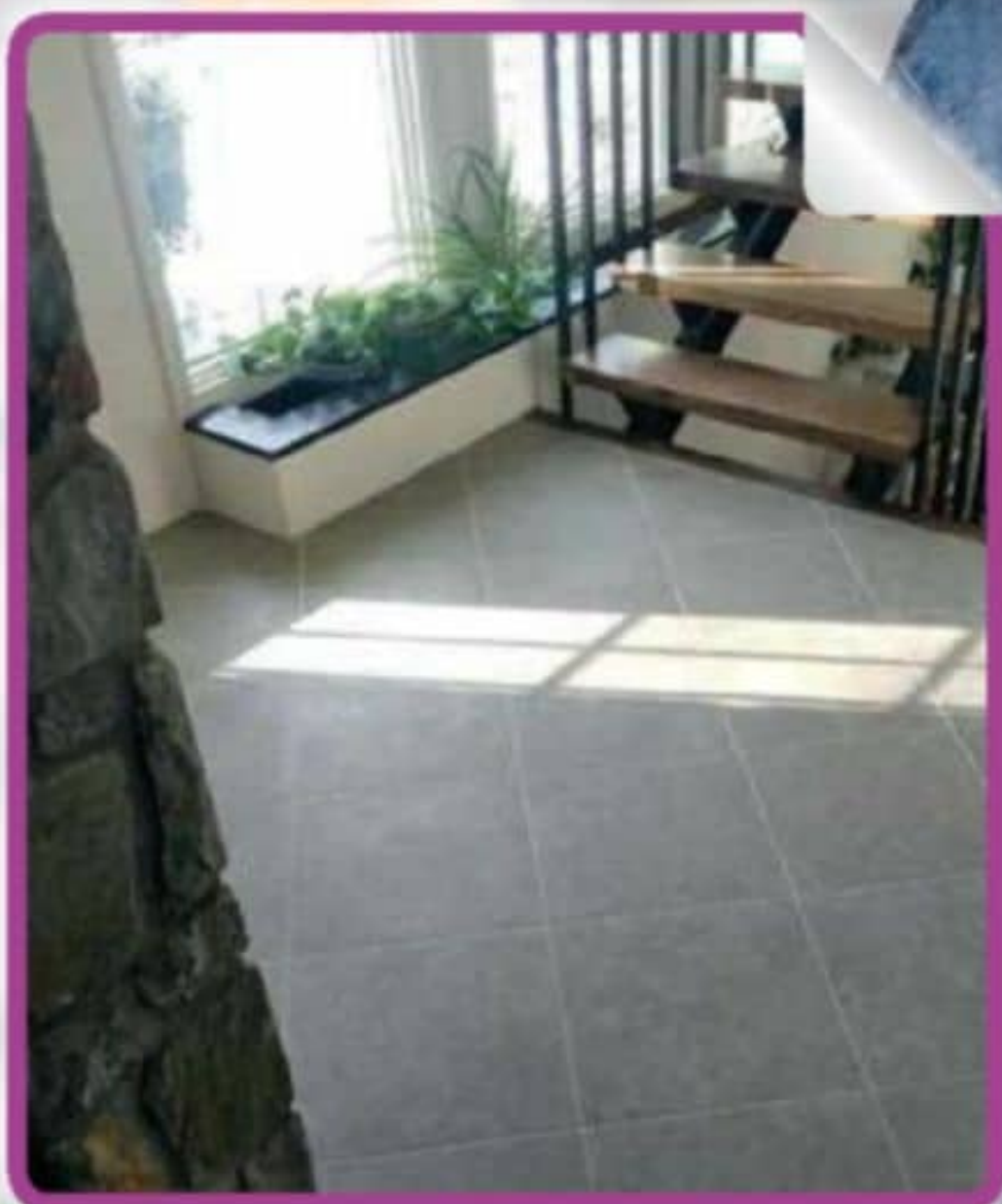
LAY VINYL FLOORING
