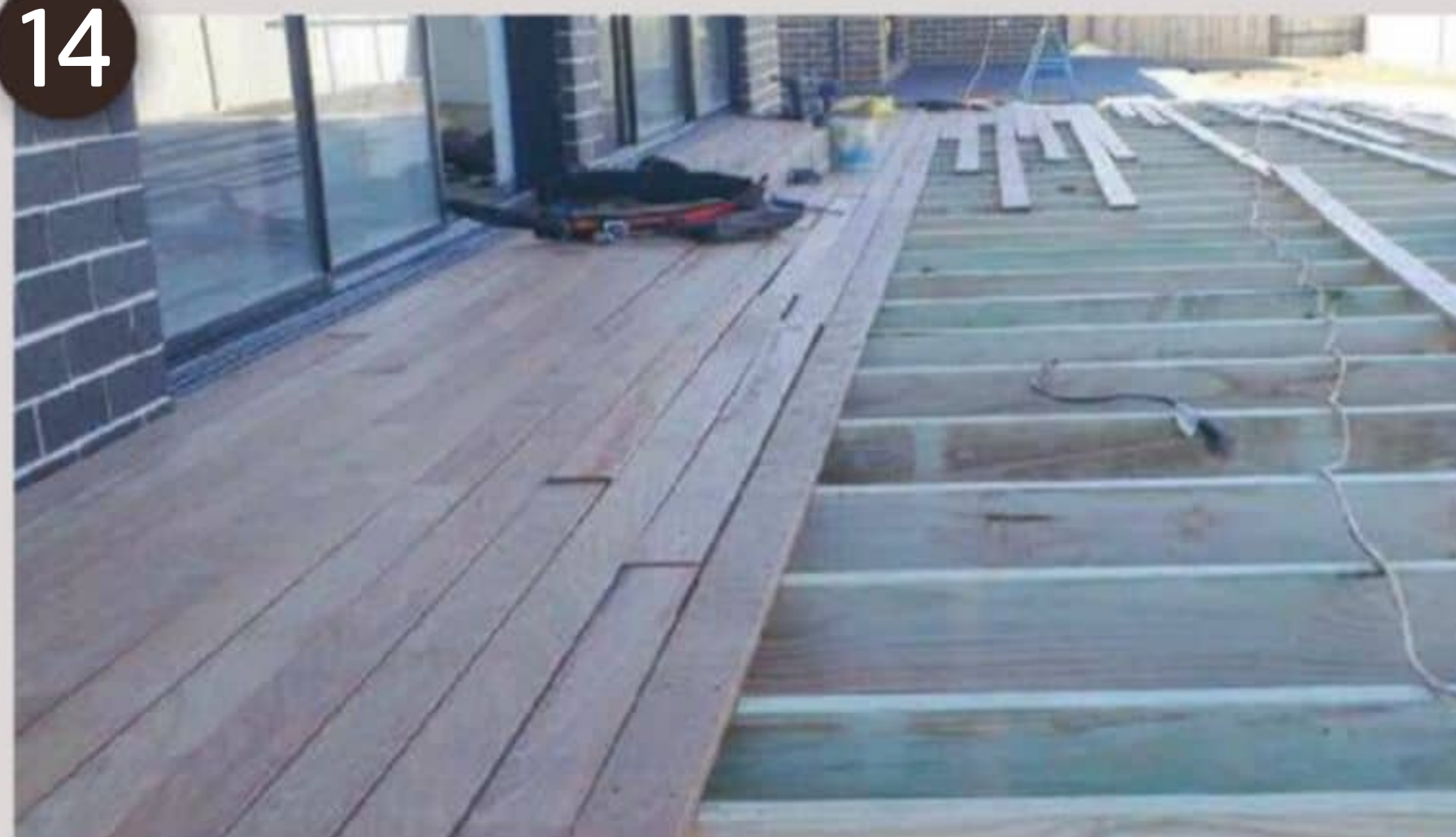
Start installing your decking boards against the house
