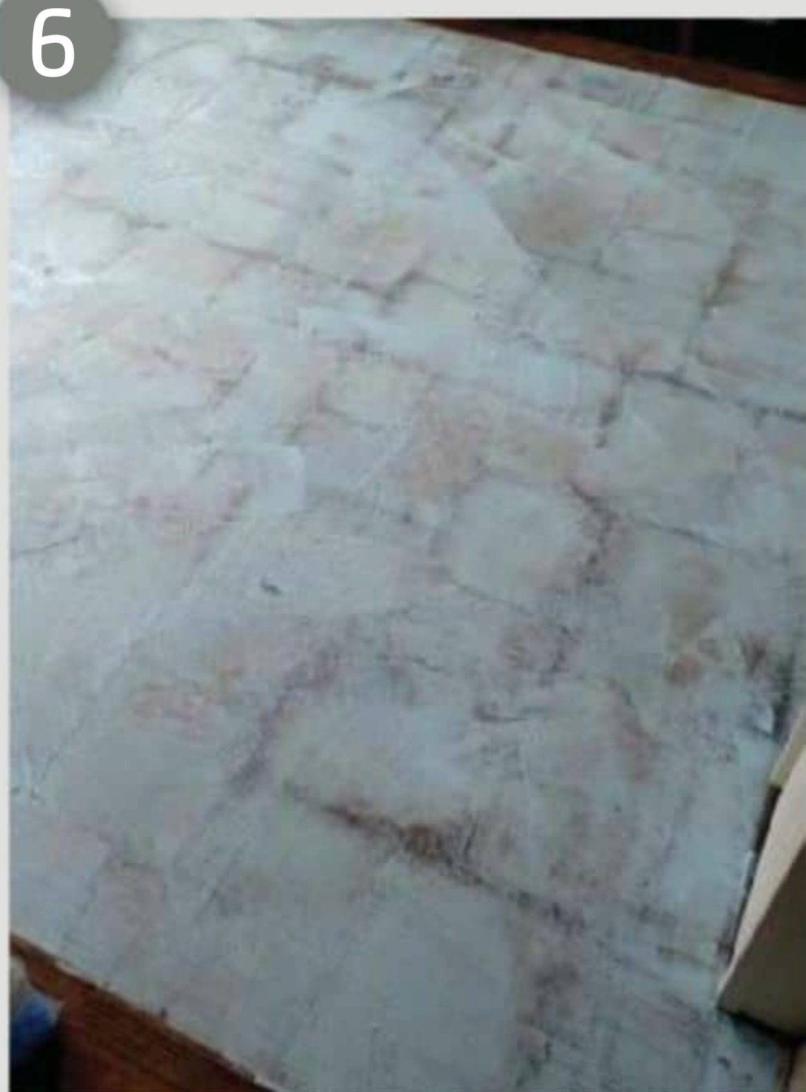
Trowel on the adhesive with a very fine notch trowel
