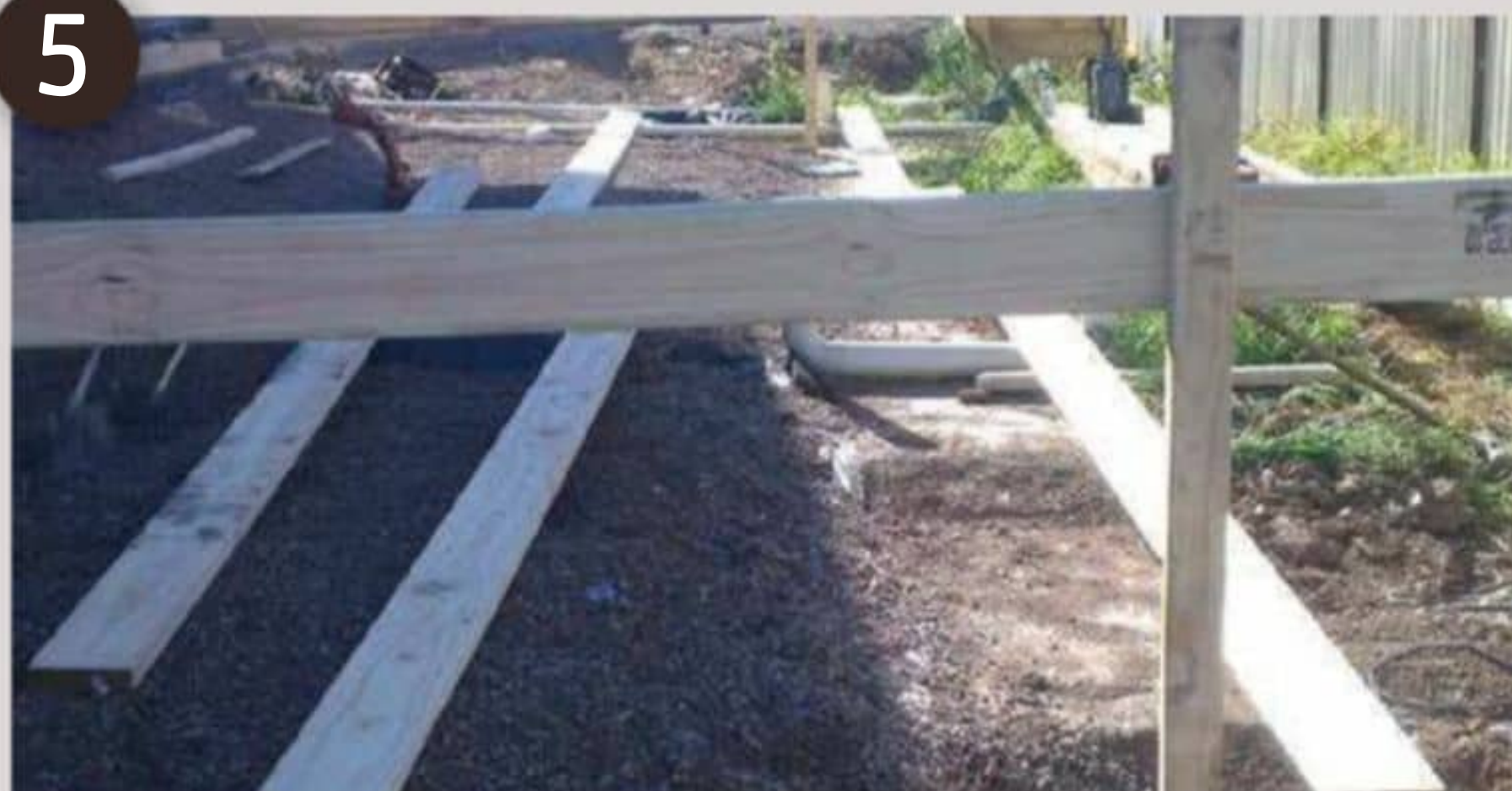
Using a level make sure you level the joist and use an offcut of timber to support the other end
