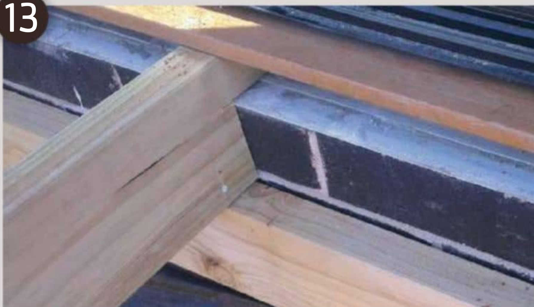
Trim your wood to fit where necessary
