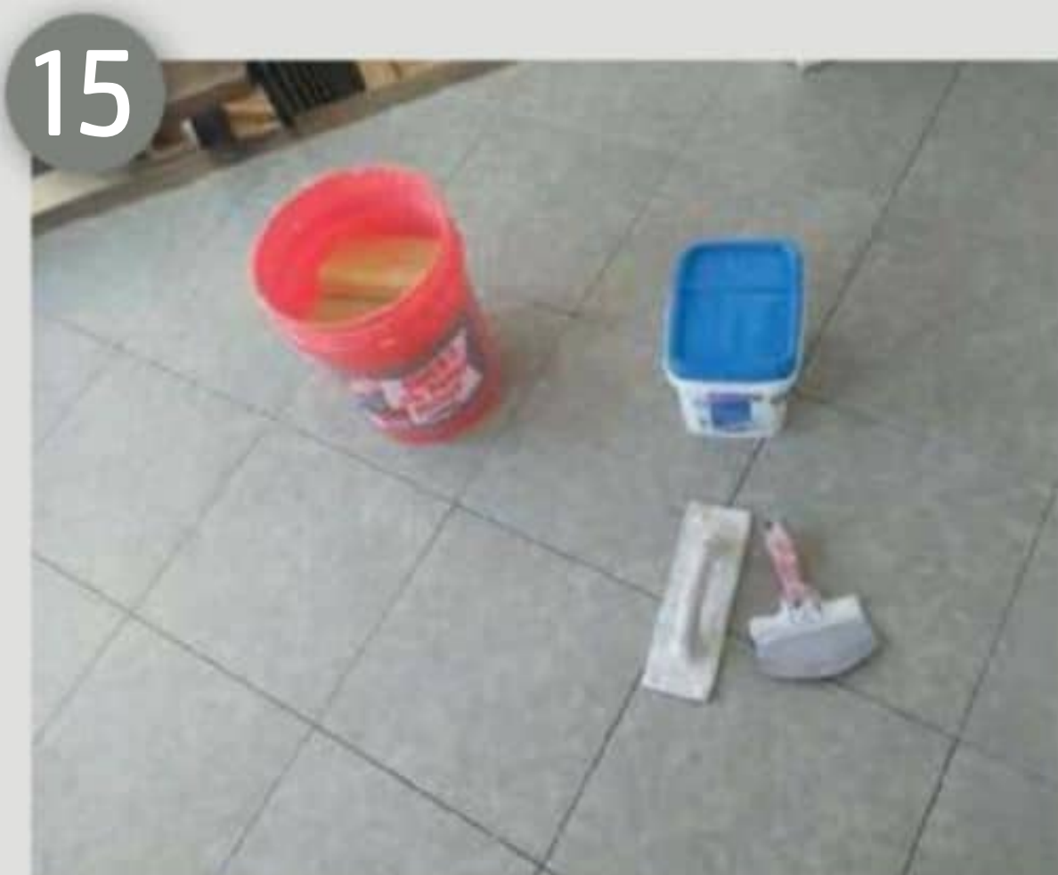
Grouting LVT is very similar to grouting ceramic tile
