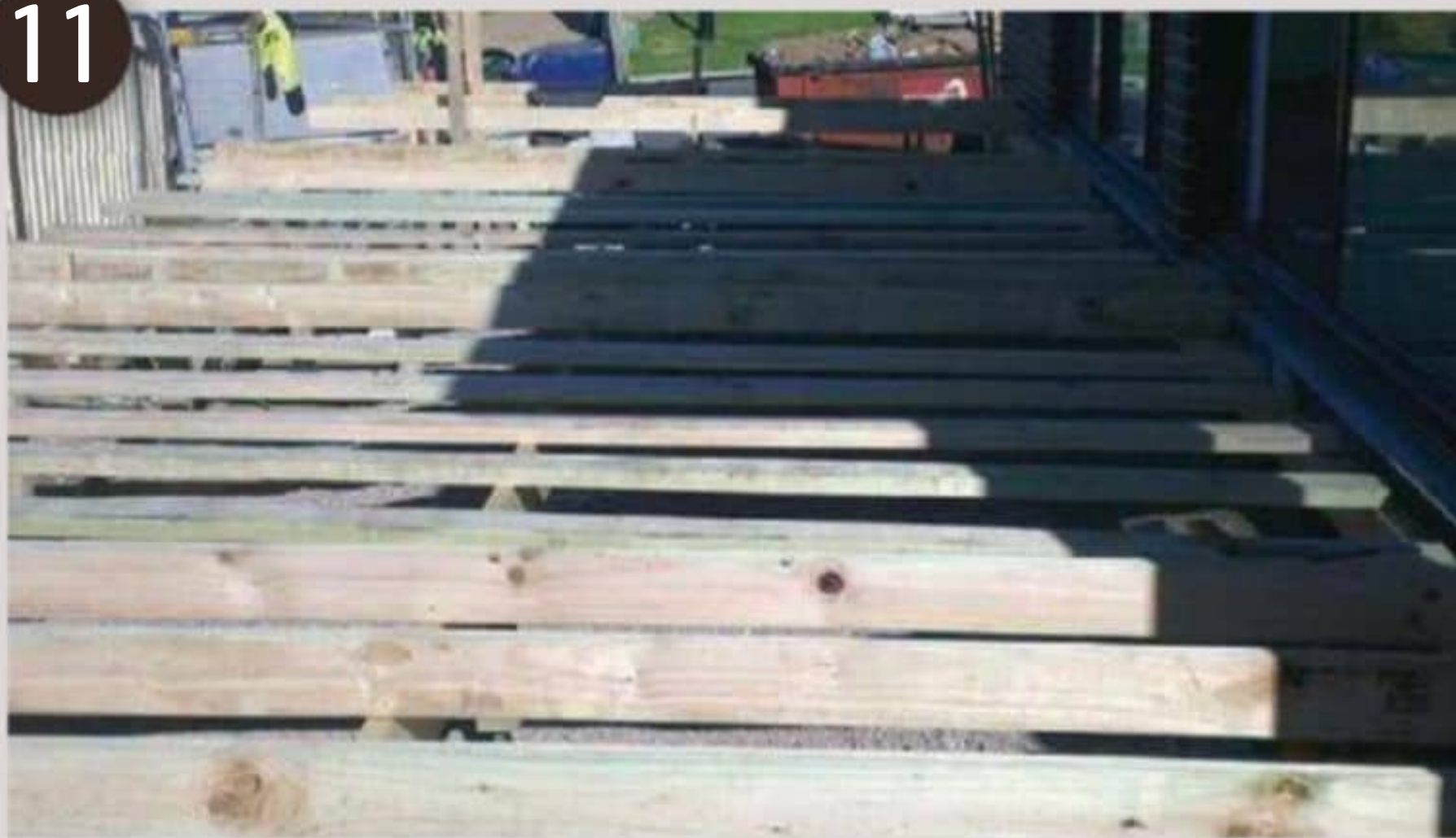
Install all your joists at the required spacing
