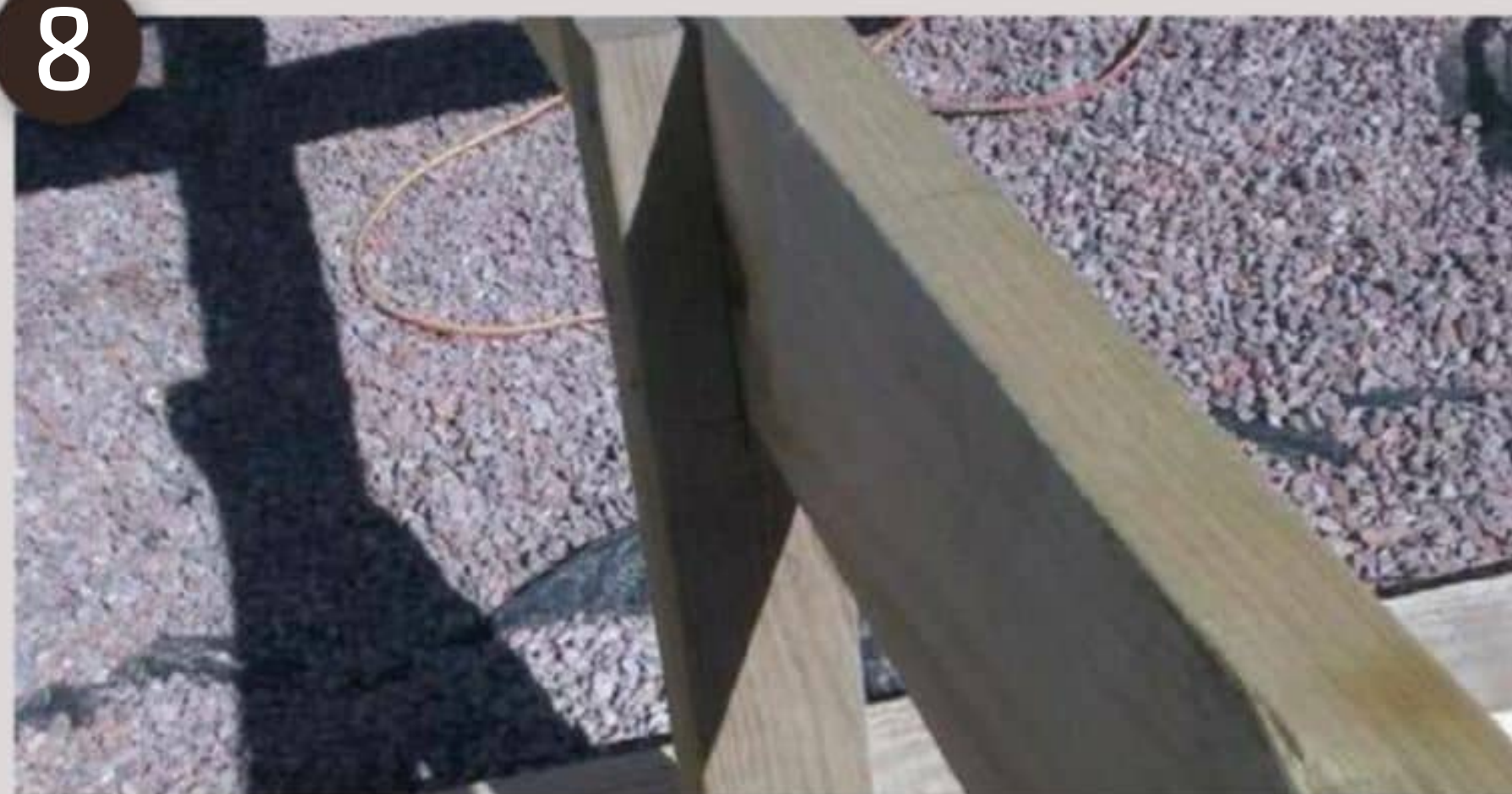
The size of your deck and the size of your wood will determine the distance between your bearers
