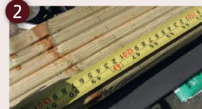
Using a standard 2.4m long plank measure 1.2m with a tape measure
