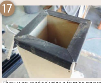
These were marked using a framing square and paint pen, and cut using a portable bandsaw
