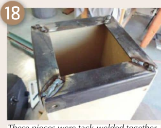
These pieces were tack-welded together, and then removed from the form to receive a full bead weld on each joint
