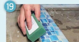
Now sand the inside and the outside glass edges with the diamond grit sanding blocks
