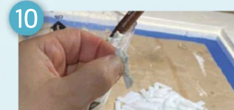
The thin-set should squish about part way up the piece
