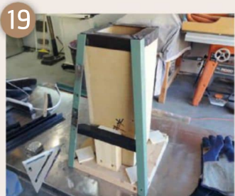
Pieces of iron were now cut to create a footrest/lower frame support for the stool
