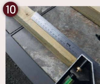
The upper shelf retainers are cut into two 18cm lengths
