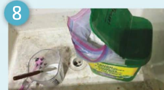
Mix the thin-set mortar
