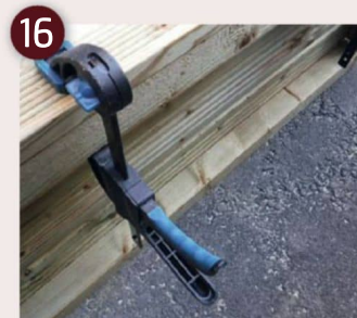
Clamp and measure and insert pilot holes
