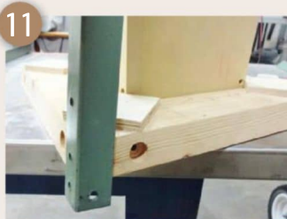
To mark these, the corner of the form was hung over the edge of the table and the metal held in place as shown
