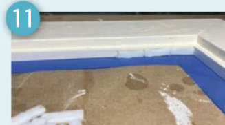
Place the next piece down trying to leave uniform gaps
