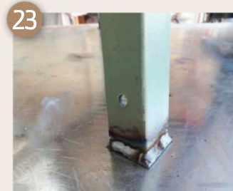
Tabs made of scrap metal were welded to the bottoms of each foot as well
