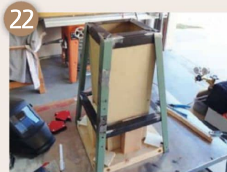
The footrest/lower support piece was held in place with support blocks on the form with the legs and stool top piece
