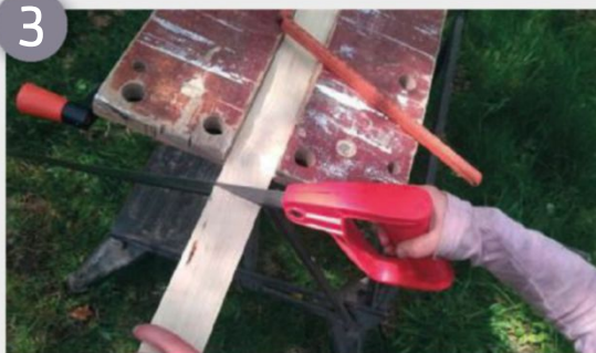
3 Saw the beams
