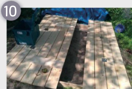
Create a small overhang, so you create some margin for error
