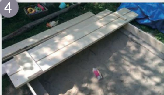
4 Glue and screw the shelves in the right place
