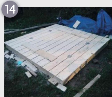
Close the lid and use a jigsaw with rails to cut the sides of the lid
