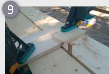
I used a wooden peg as distance holder between the shelves
