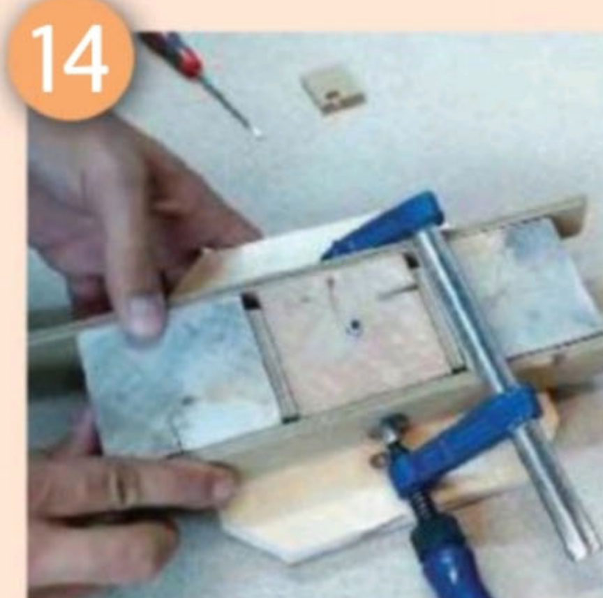
I wanted there to be a 7mm gap between the blocks, so I used 7mm spacers
