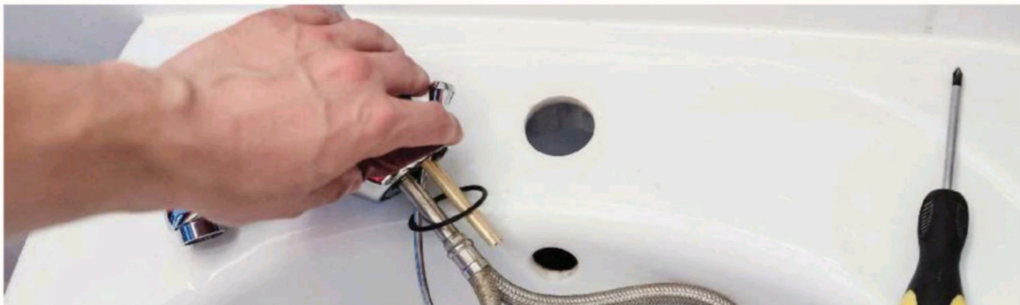
Replacing a tap is a job most DIY'ers can accomplish
