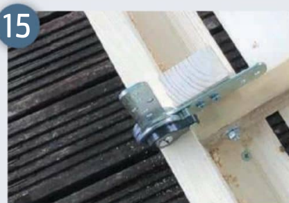
15 I bolted and screwed the end two hinges straight to the existing end pieces of timber
