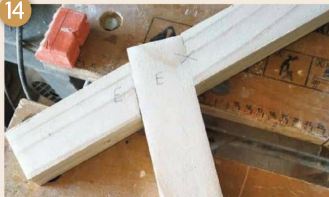
Fig. 14: Marking-up each fitting joint
