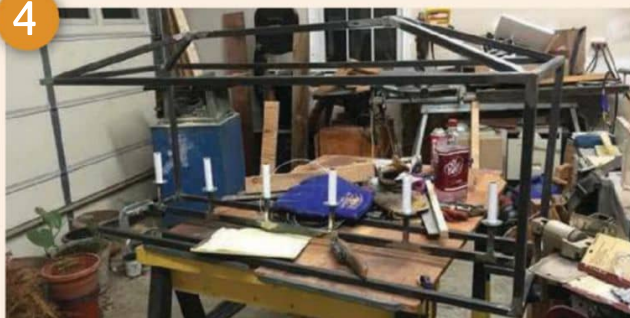
With the light bar complete, I welded it into the frame
