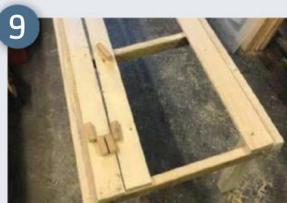
9 The slats are cut to size on the chop saw, and placed individually on the framework
