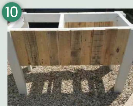
10 The pallets were used as rustic cladding
