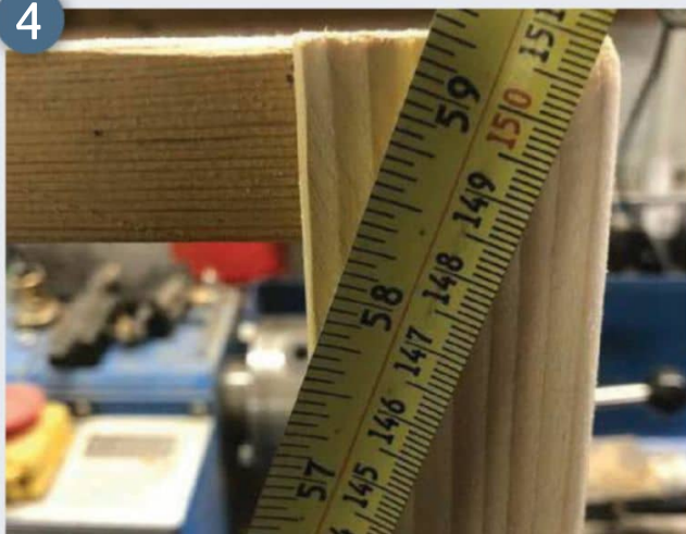
The framework is for the horizontal slats
