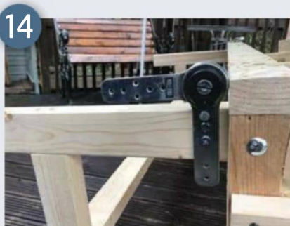
14 I found ratchet hinges to use for the footrests
