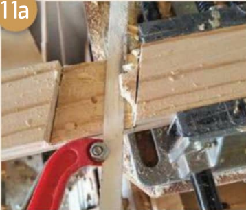
Figs. 11A and 11B: Using a hacksaw and using a coping saw
