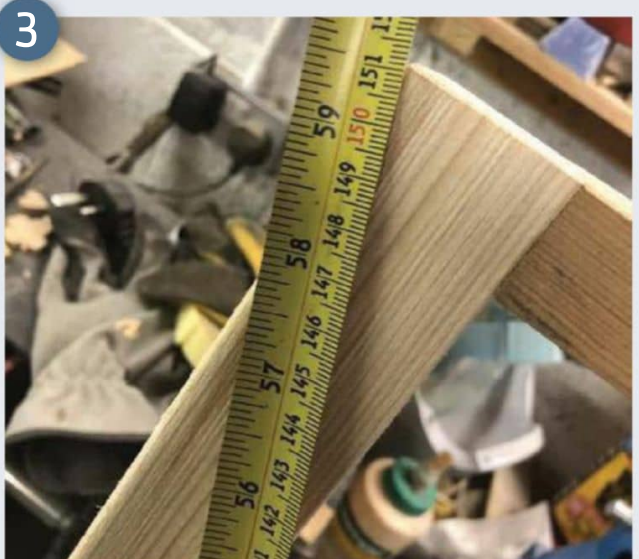
Check the diagonals to ensure the framework is square
