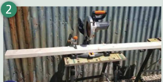
Next step was to build the four legs
