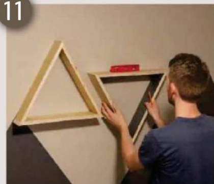
Measuring and marking for attaching to the wall
