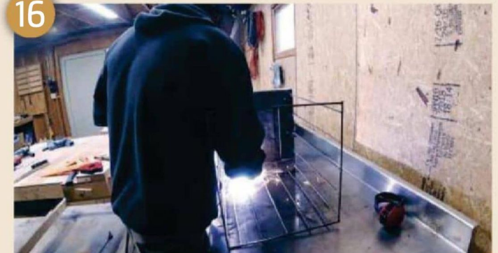
Weld one piece of 500mm on every side to keep it level and square
