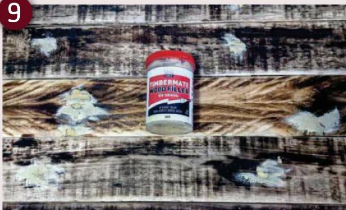
I grabbed some filler from my garage shelf and got the holes filled in and sanded off
