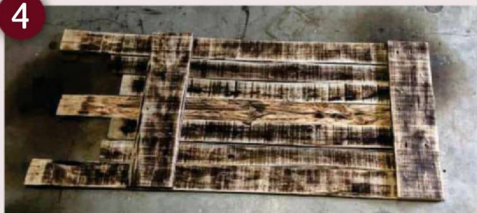
Using screws I fixed together the table top with a couple of cross braces on the underside
