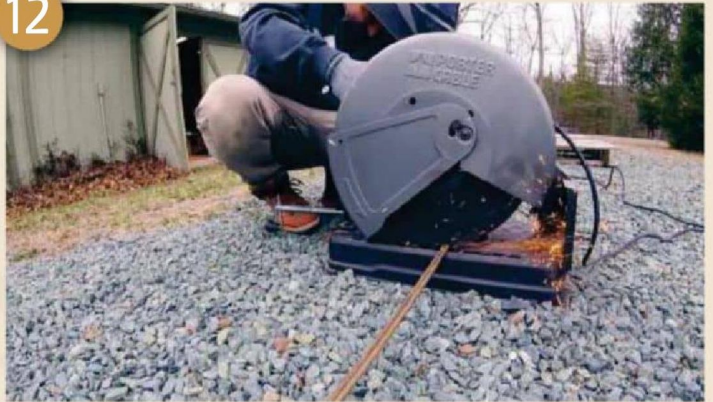
Cut your steel rod to size
