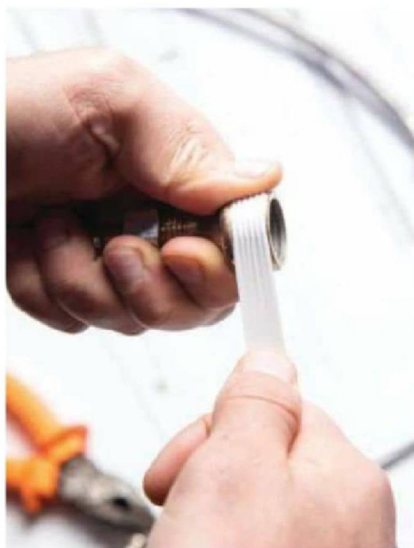
PTFE tape to seal for leaks
