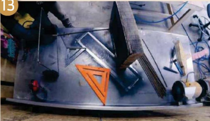
After your pieces are cut it's time to weld the cage
