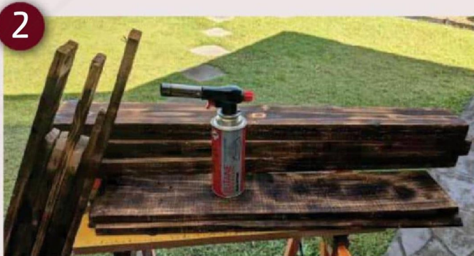
Using a butane torch I lightly burnt the surface of all the pallet wood
